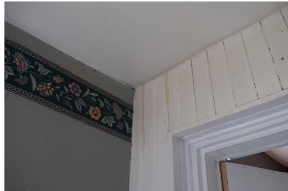
Photo 38: Plaster walls and wooden paneling on former exterior wall in rear addition, looking southwest
