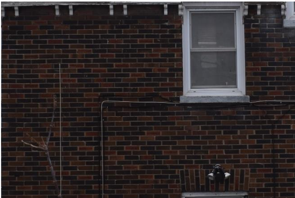
Photo 3: Brick bonding and soldier course, looking north
