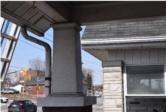
Photo 5: Tapered, square wood support columns, looking northwest
