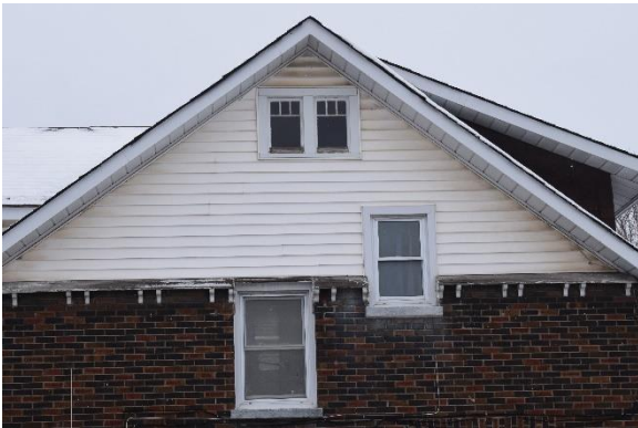
Photo 15: Wood frame windows in gable peak and wooden trim on south façade, looking north
