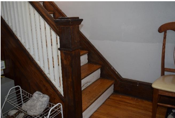
Photo 41: Staircase with original newel post, banister, and wooden trim leading to the second storey, looking southeast
