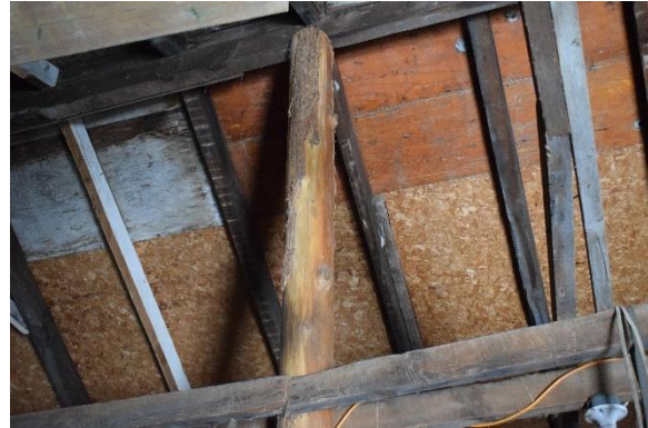
Photo 39: Machine cut beams and timber centre post, looking west
