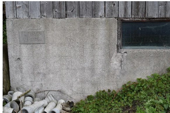
Photo 5: Representative poured concrete foundation photo, looking east
