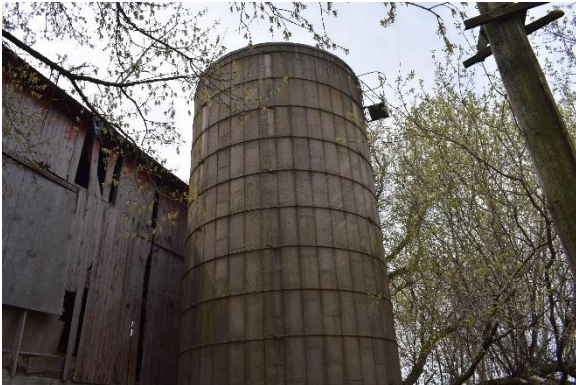
Photo 30: Cast-in-place concrete silo, looking south
