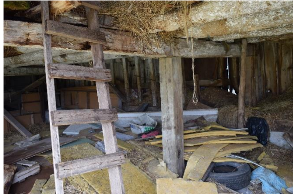
Photo 23: Hand hewn and log posts and beams and ladder, looking north
