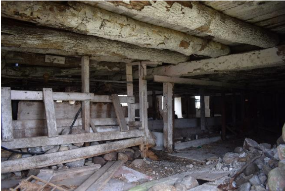
Photo 18: Lower level, showing predominantly hand hewn and log area, looking south
