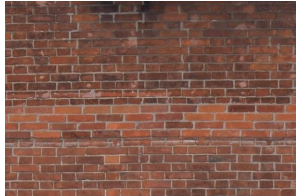
Photo 7: Flemish brick bond and four rows of stretcher bond bricks between the upper and ground storey, front (south) façade, looking north
