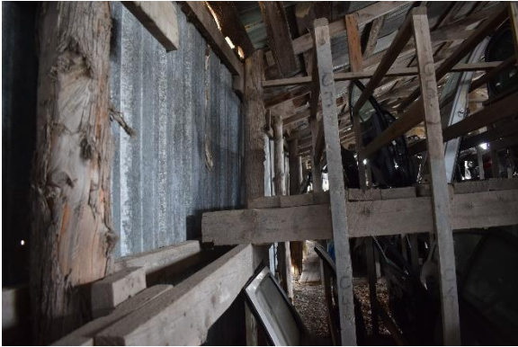
Photo 96: Interior showing mix of machine cut and log beams, looking east
