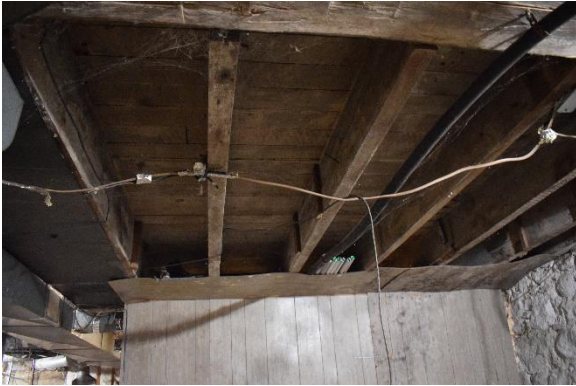
Photo 44: Hand hewn and machine cut beams, looking east
