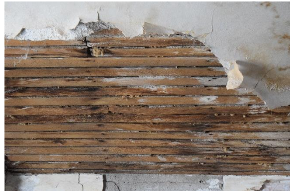
Photo 73: Exposed lath and plaster, looking east
