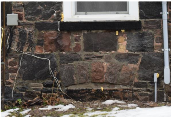
Photo 16: Basement level stone voussoir, looking west
