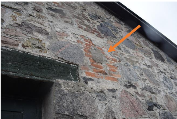
Photo 22: Brick infill (denoted by arrow), looking south
