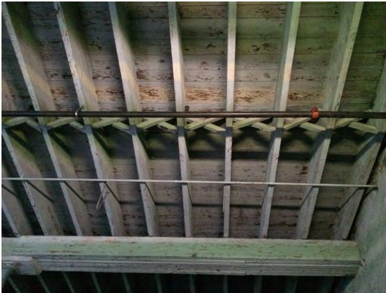
42. Part 1. Detail of wooden floors/ceiling of the second floor, viewed from ground floor interior. (Source: ERA Architects)
