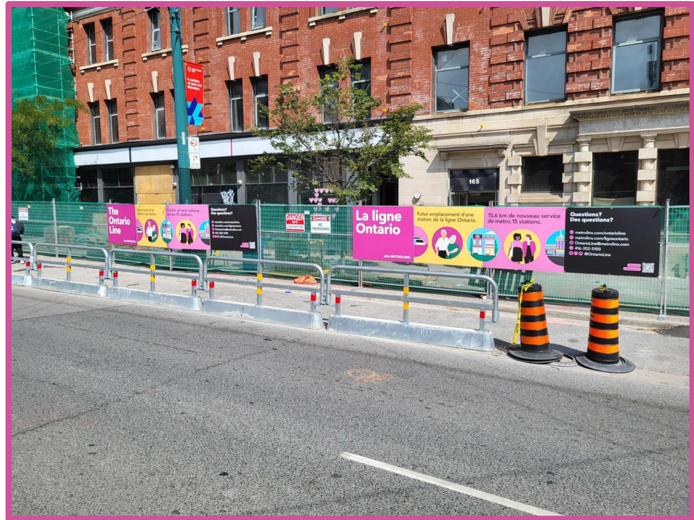
Metrolinx temporary project signage installed along Queen Street West.
