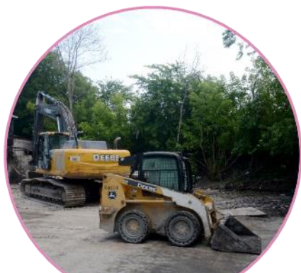
EXCAVATOR AND LOADER
