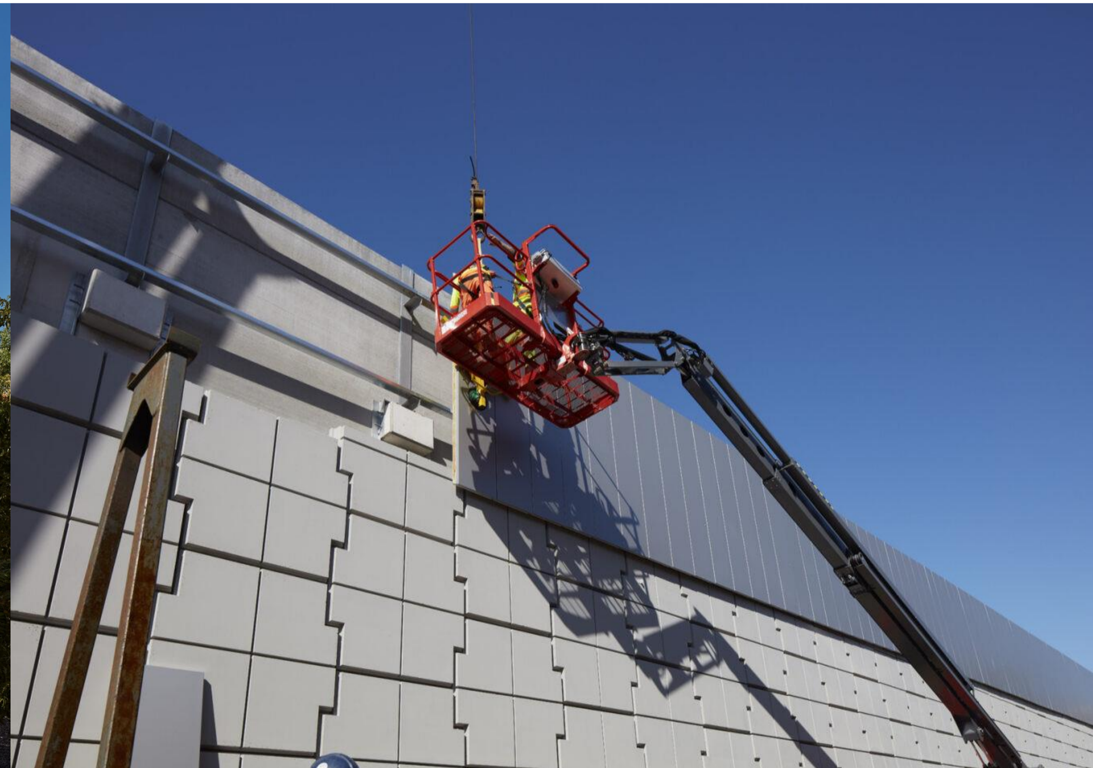
Cladding installation on the Elevated Guideway
