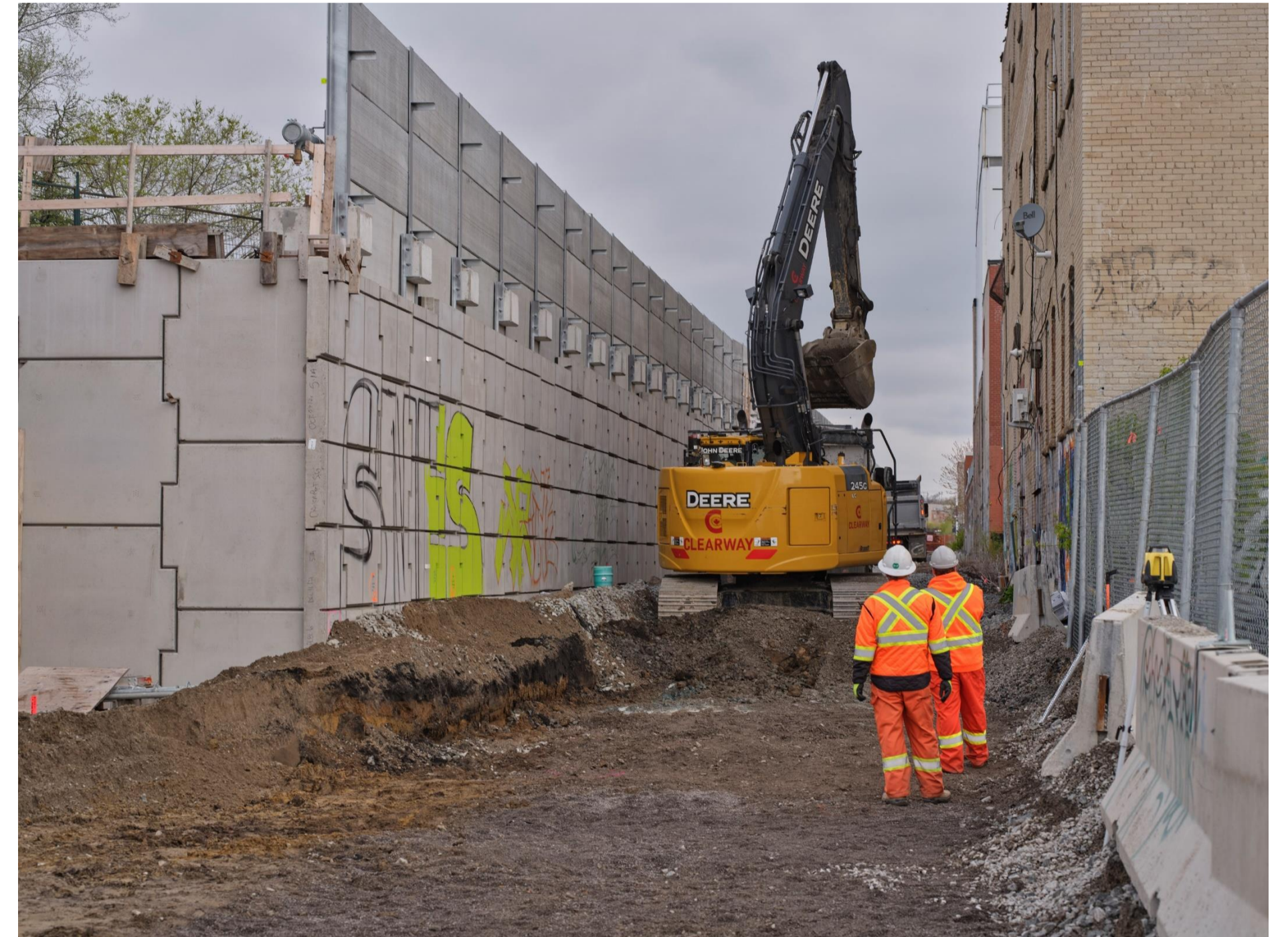
Excavation for drainage installation beside the S-MSE walls
