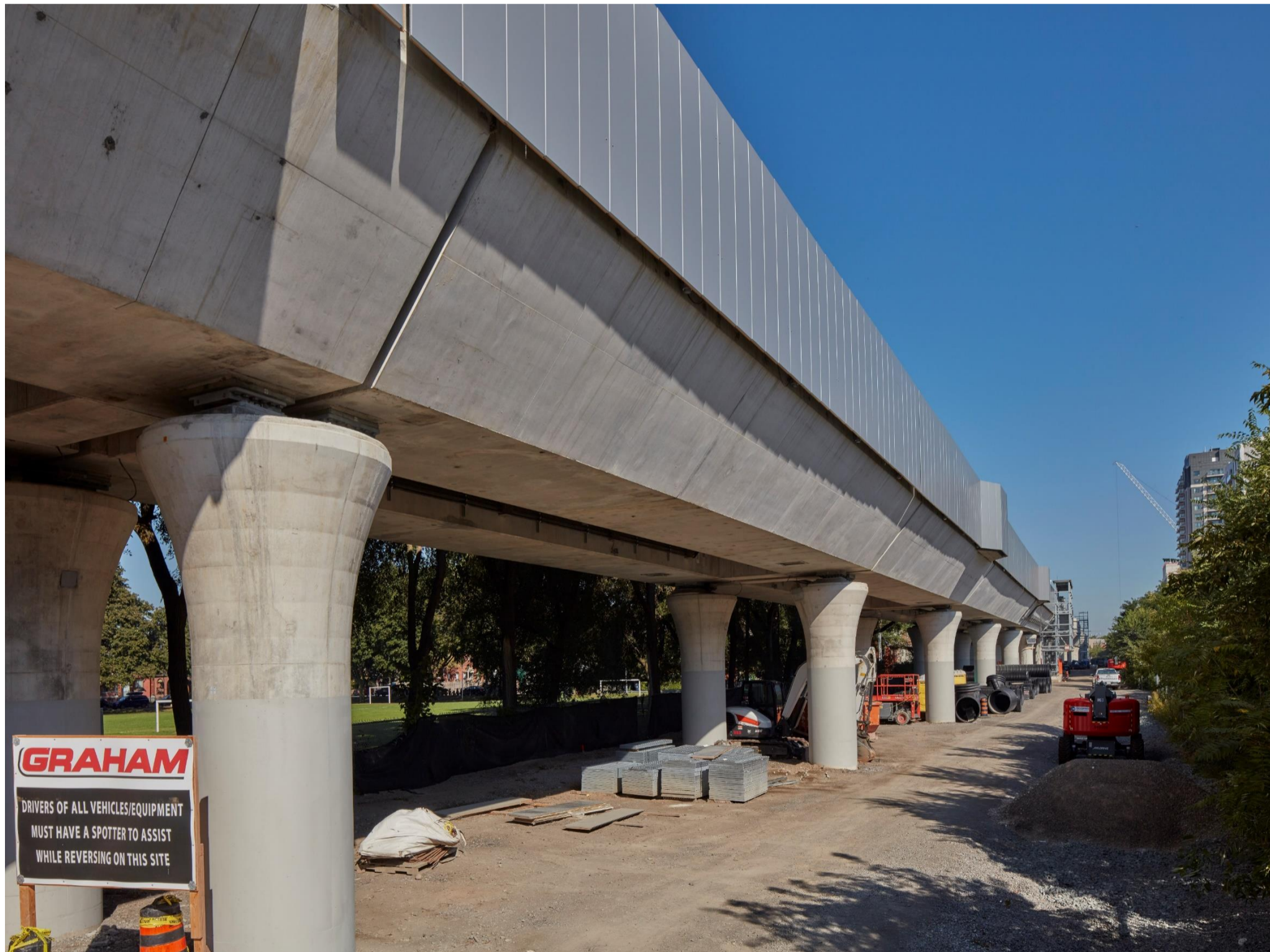
Cladding installation on the Elevated Guideway
