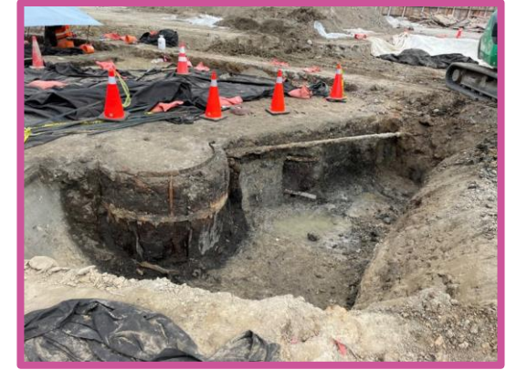
Wooden barrels from a water cistern at the Hamilton/St. Lawrence Foundry Site (AjGu-124)
