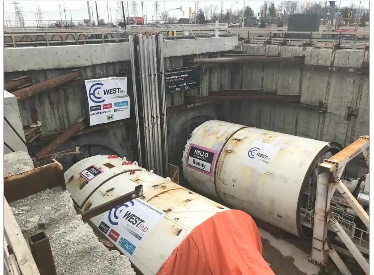
Photo courtesy of Metrolinx Eglinton Crosstown West Extension project.
