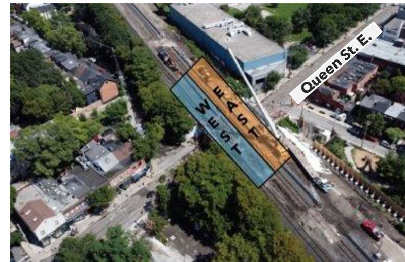
Shoring wall at Dundas St E bridge
