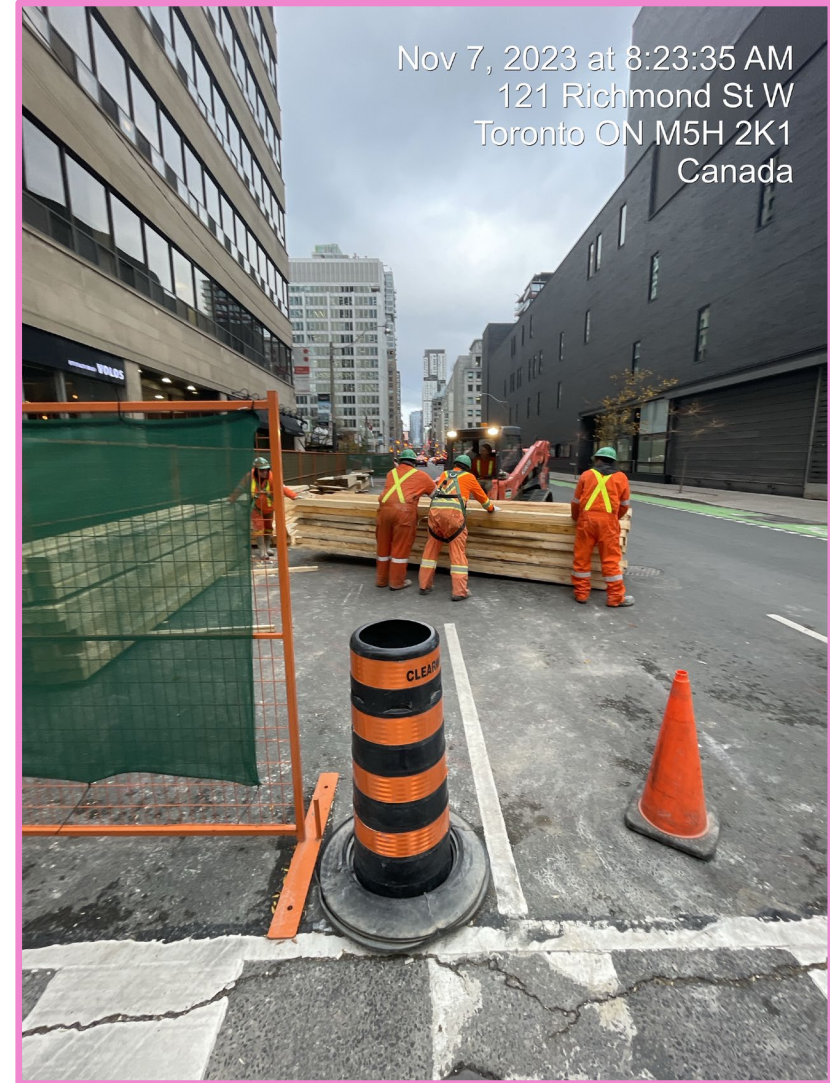
Hoarding and fencing staging facing southbound at York Street.
