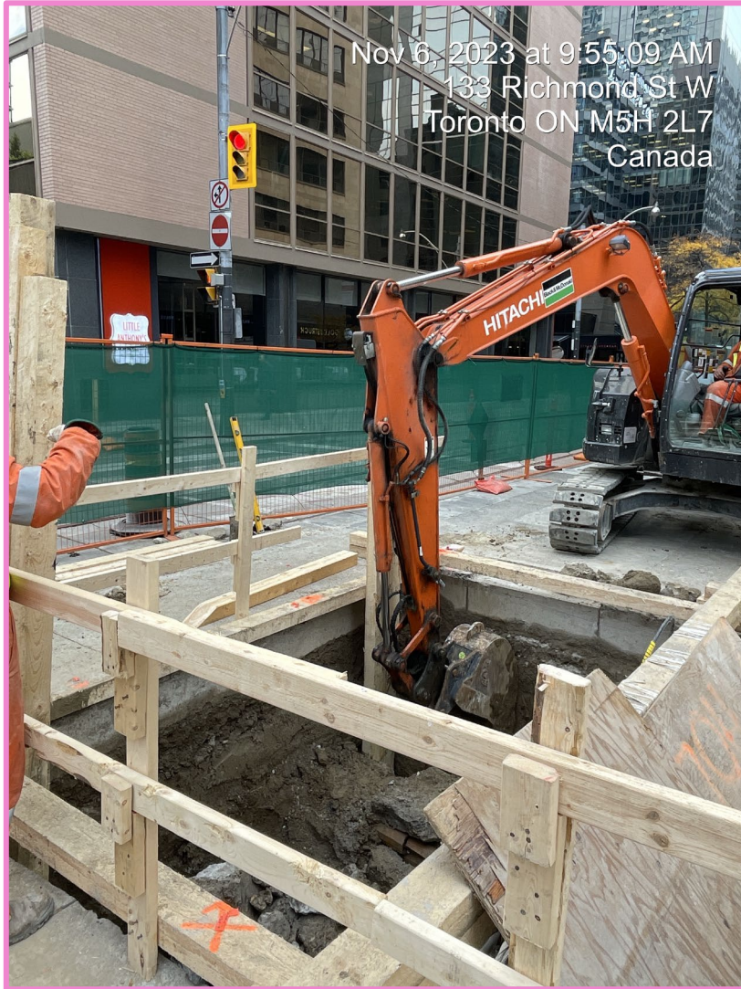
Chamber construction at Richmond Street and York Street intersection
