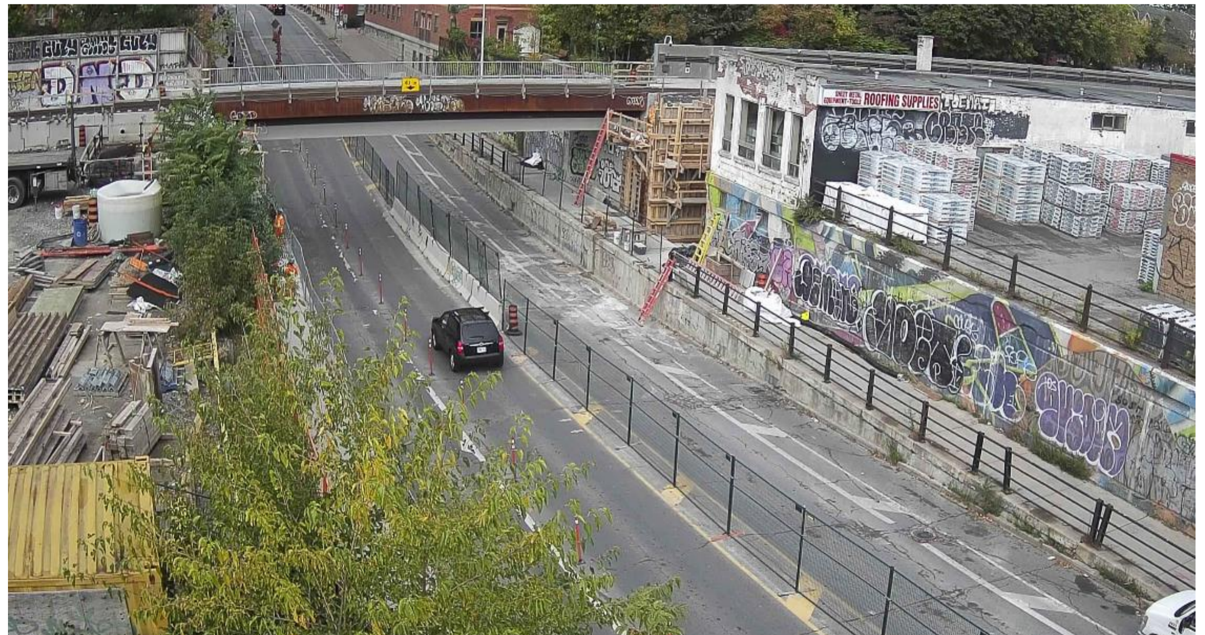
Bloor St Bridge and partial closures
