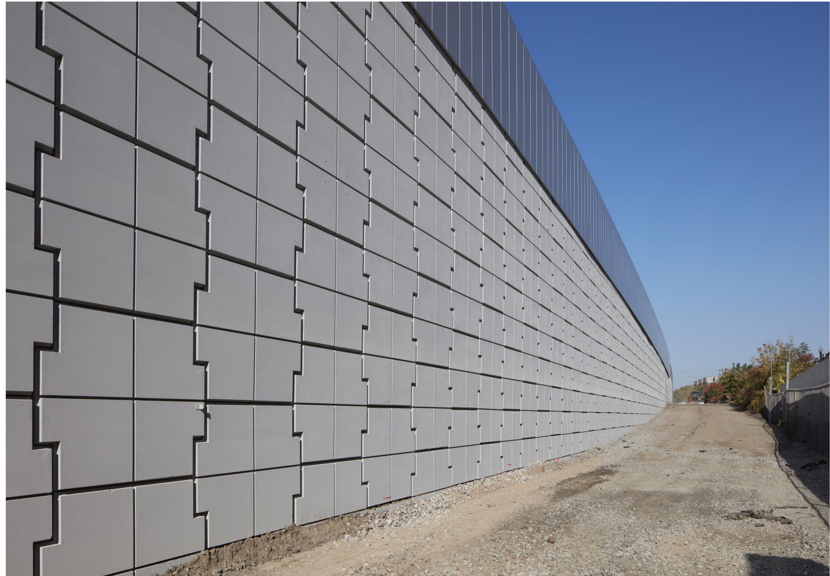
North MSE wall construction
