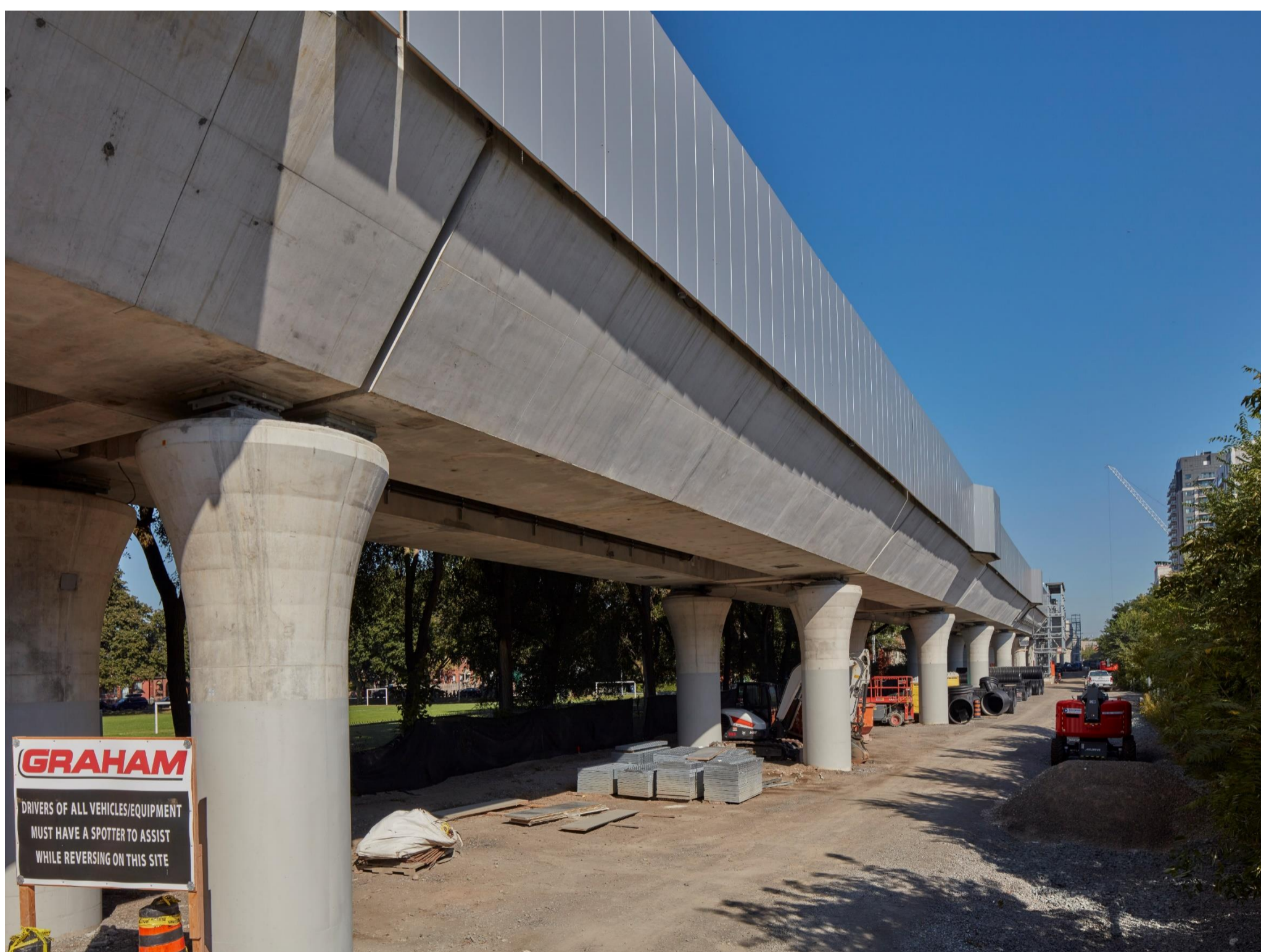
Cladding installation on the Elevated Guideway
