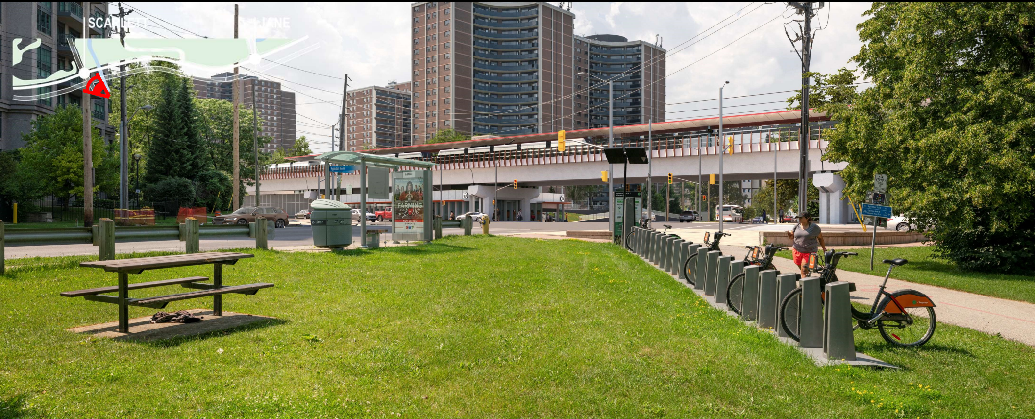
Scarlett Road (looking north) - 30 years post construction
