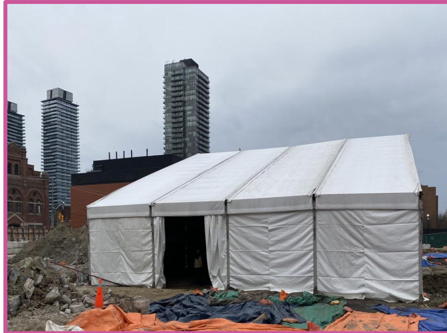
Tent facing Southwest
