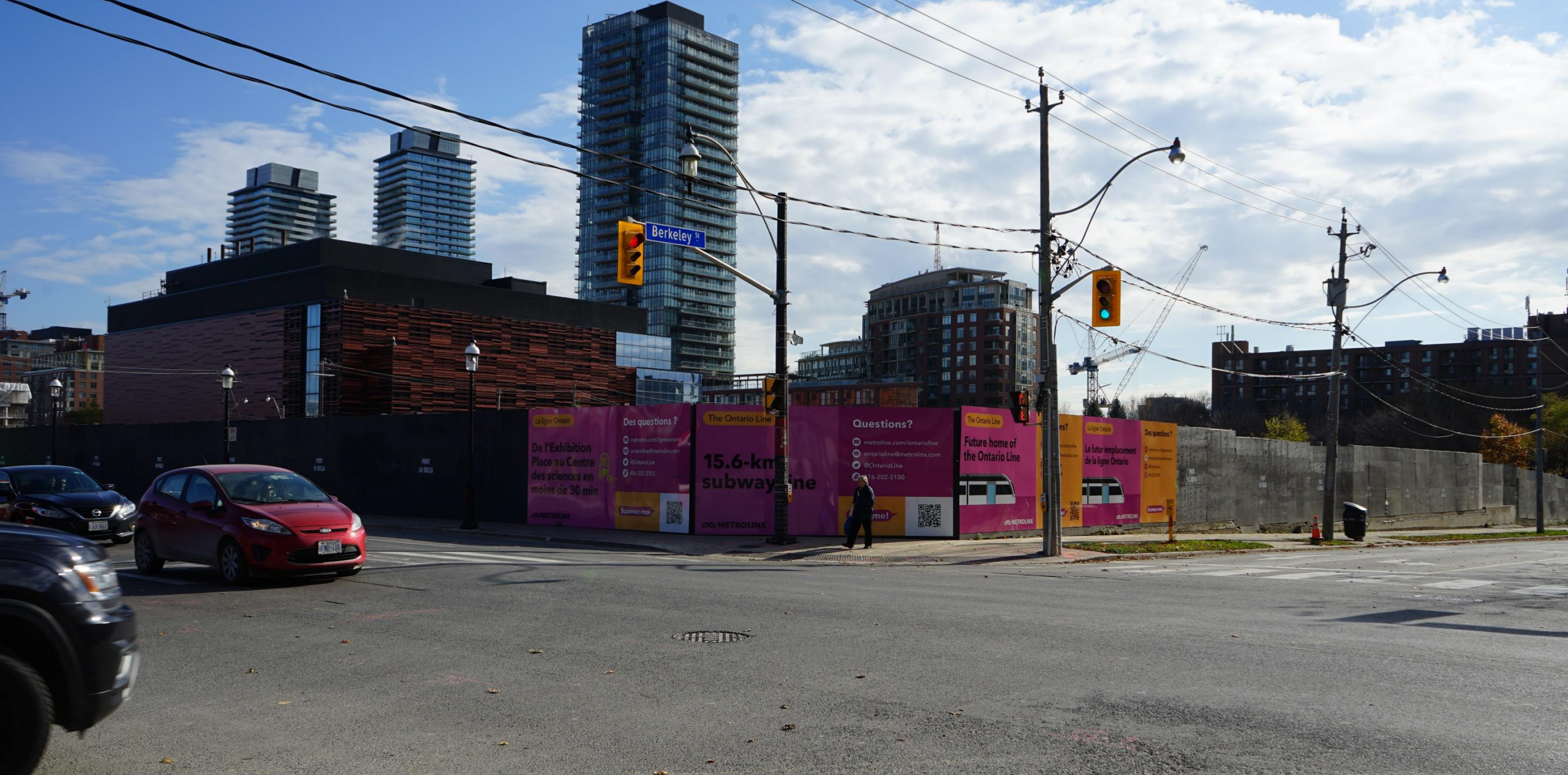
Future site of the South entrance
