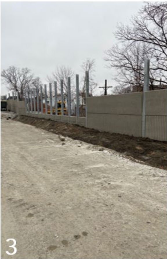
3 & 4. Noise Barrier Wall Construction
