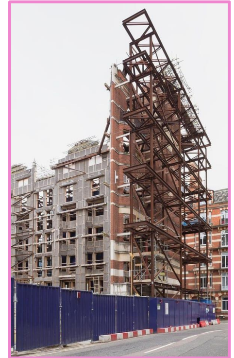
Visual example of retention towers
