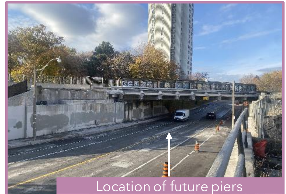
Shoring wall at Logan Ave.
