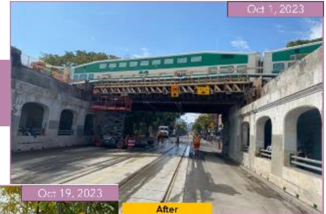
Queen St E Bridge demolition
