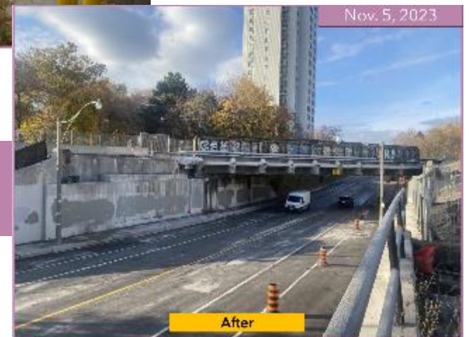
Logan Ave Bridge demolition
