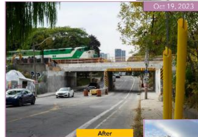
Dundas St E Bridge demolition
