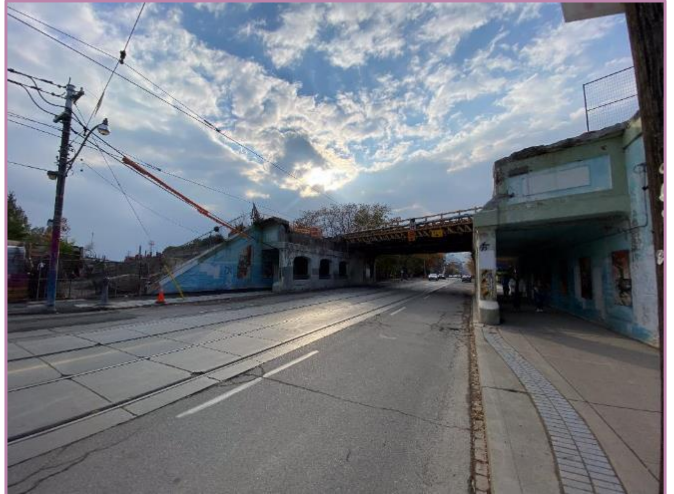
Queen Street East from the north sidewalk looking west
