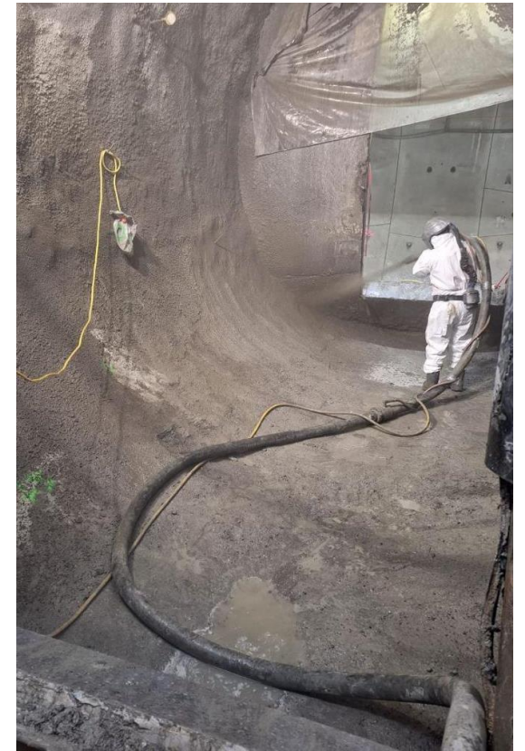
Excavation and Primary Lining
