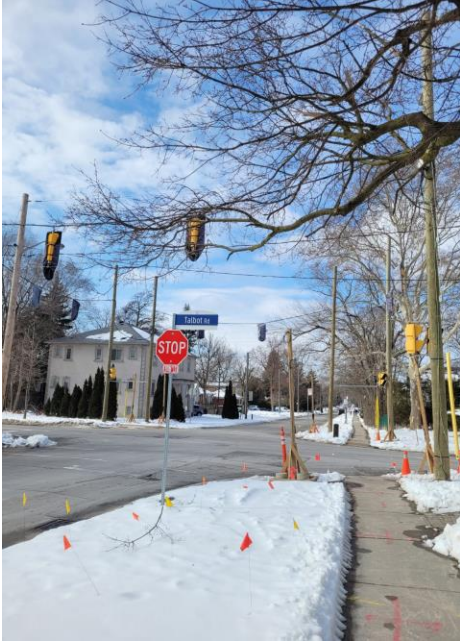
New temporary traffic signal at Hendon & Talbot under construction
