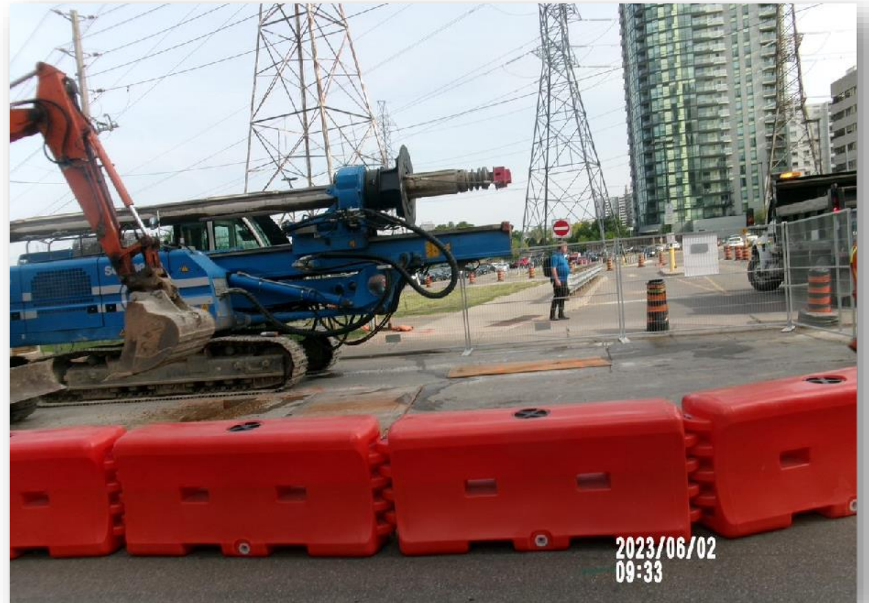
Drilling caissons
