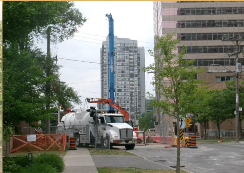
Excavation activities by earth line will allow drilling caisson to occur
