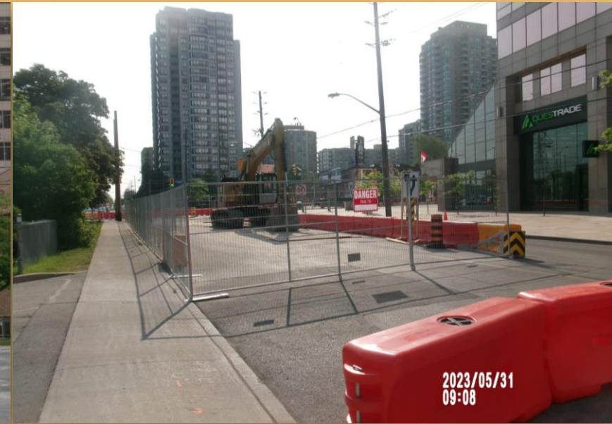
Fencing around the public walkway
