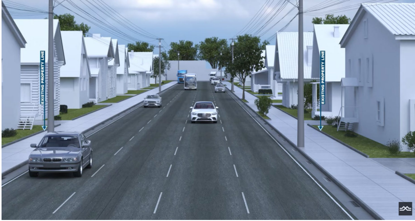
Existing road conditions.
