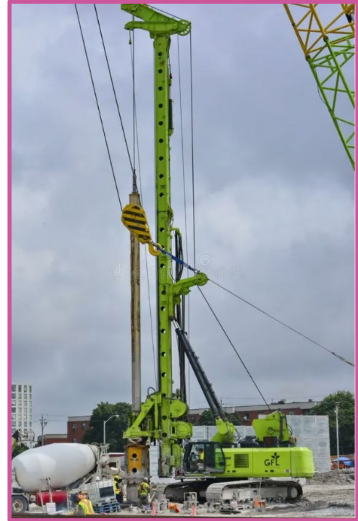
Example of a drilling machine used in piling construction
