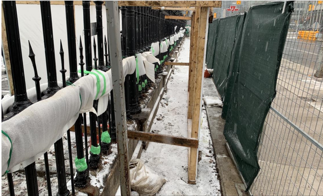
Photo Credit: Metrolinx Project Team - January 23, 2024
