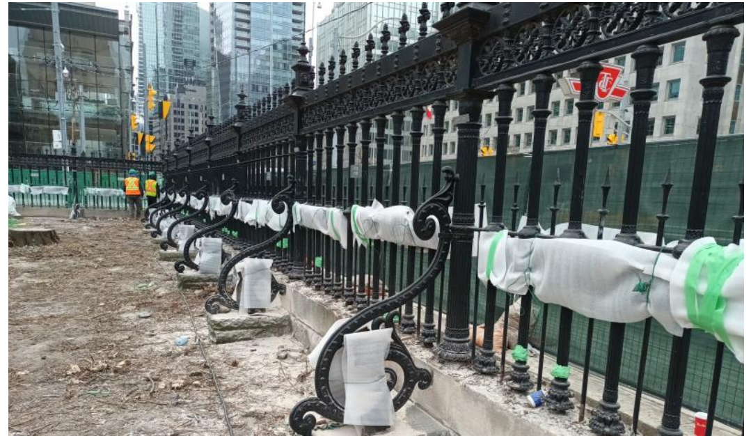
Photo Credit: Metrolinx Project Team - January 23, 2024
