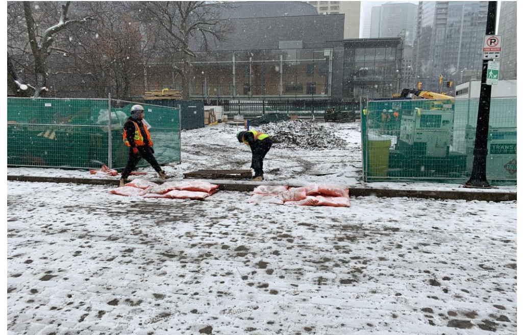
Photo Credit: Metrolinx Project Team - January 23, 2024
