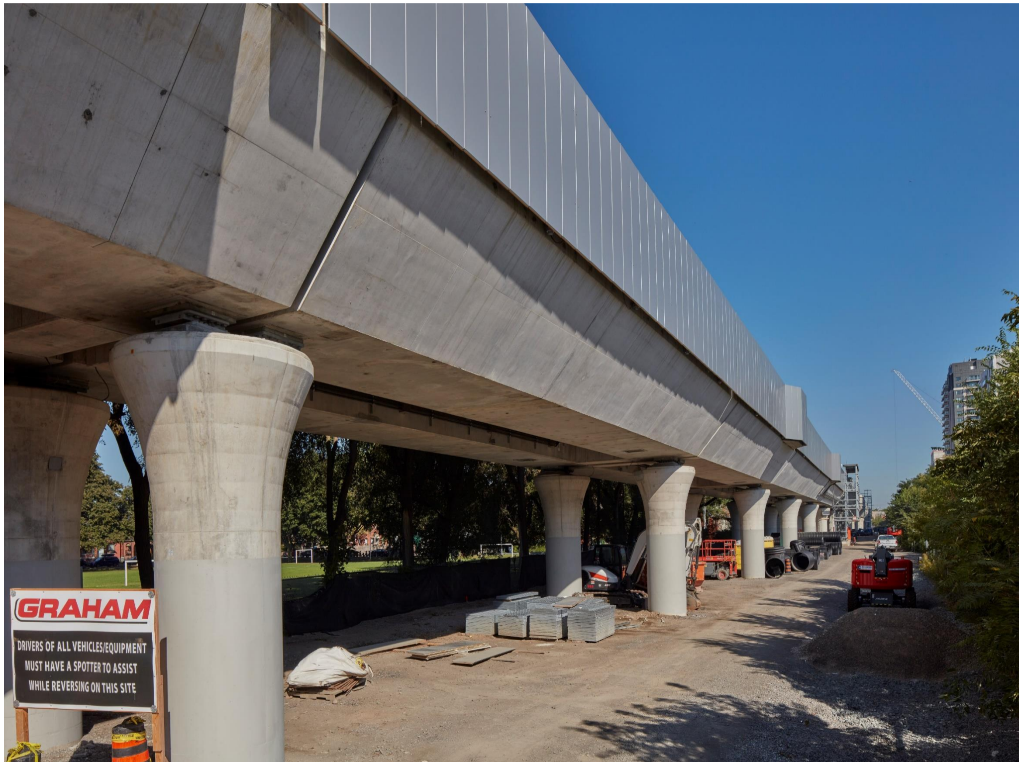
Cladding installation on the Elevated Guideway
