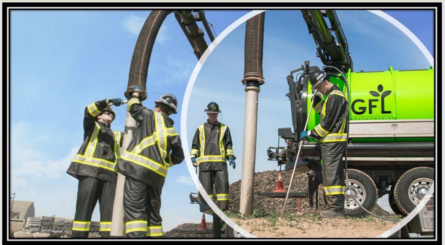
GFL crew using a hydrovac truck to expose intricate utility infrastructure as found in the Union Station Rail Corridor - East (photo courtesy of GFL)
