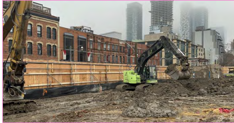
Excavator and compactor
