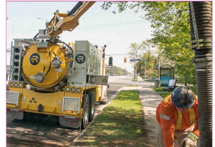
Hydrovac truck and operator
