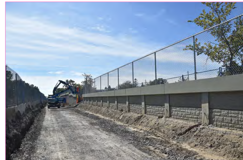
Example of a retention wall being constructed adjacent to future rails
