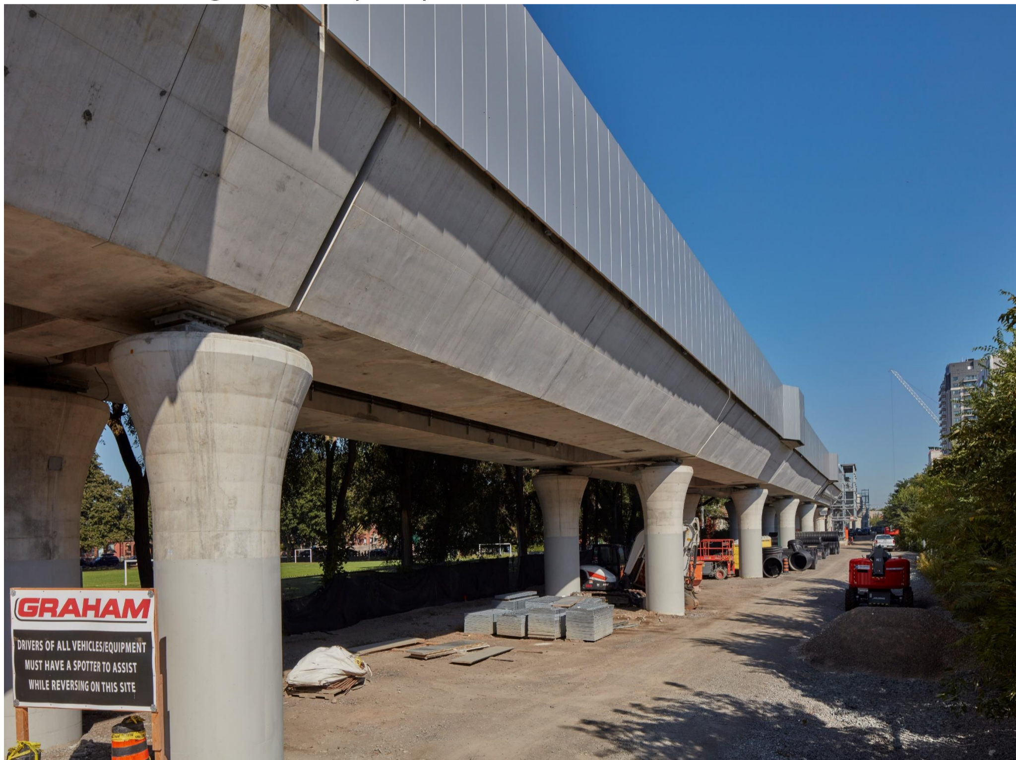
Cladding installation on the Elevated Guideway
