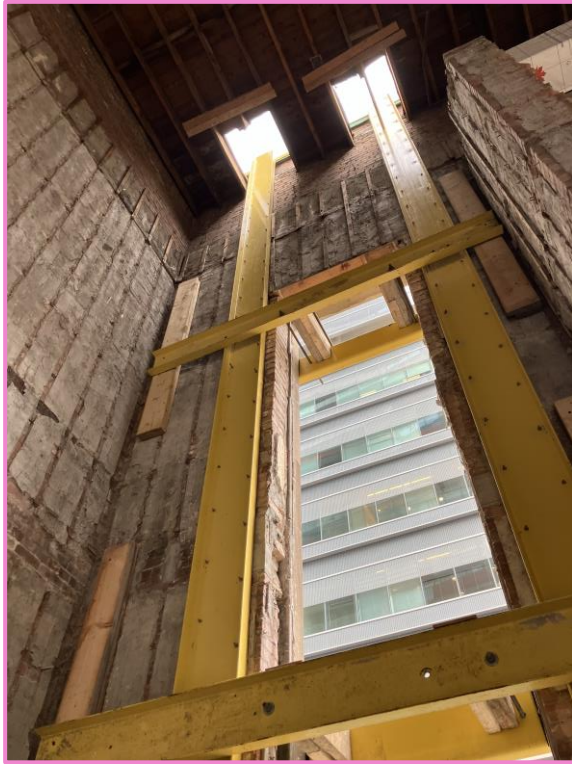
Inside view of the north façade of the building
