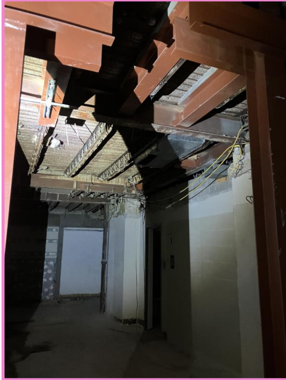
Metallic beam to support the roof top, in the basement
