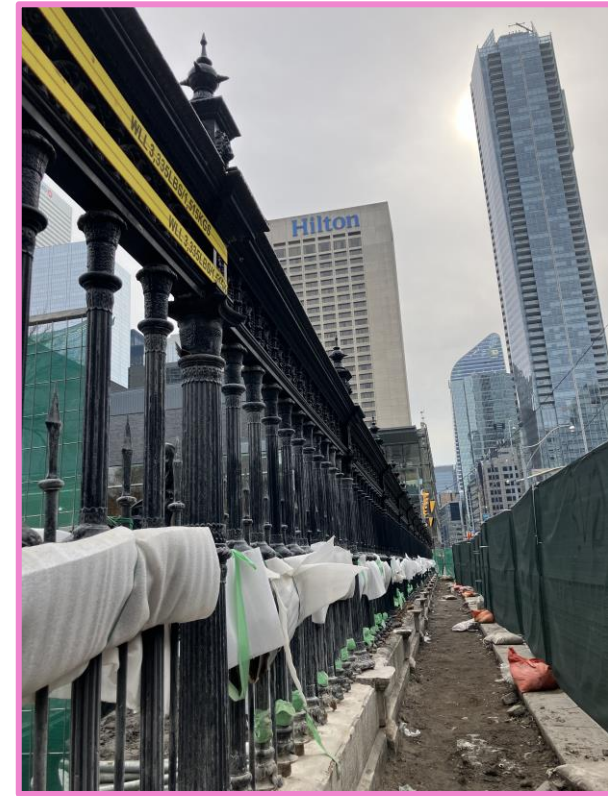
Heritage fence work along University Avenue
