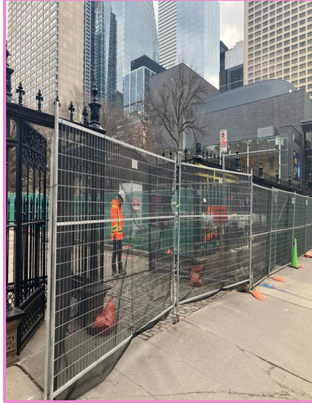
New construction gate installed, heritage gate (behind) to be removed
