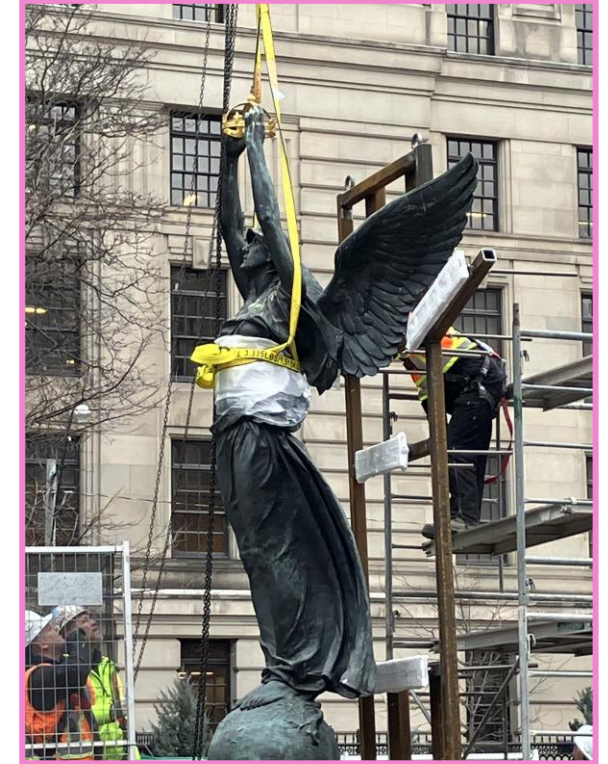
Installation of Victory Statue on transport cradle before transportation
