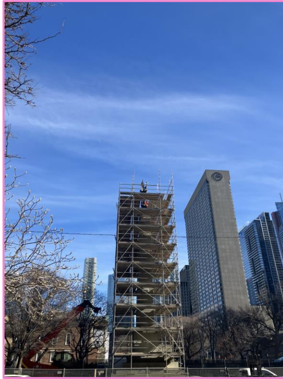
Scaffolding installed to prepare for removal of Victory Statue
