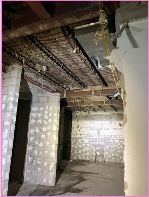
View of the basement
