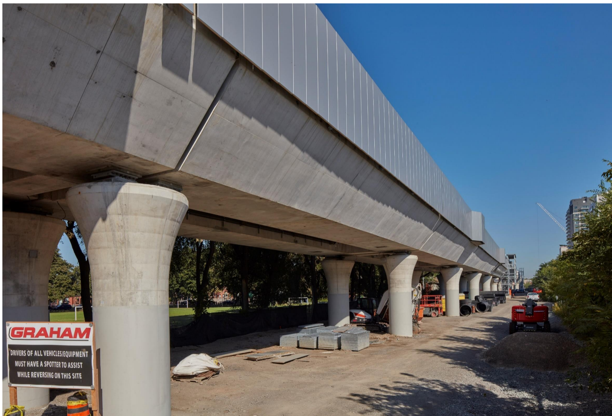
Cladding installation on the Elevated Guideway
