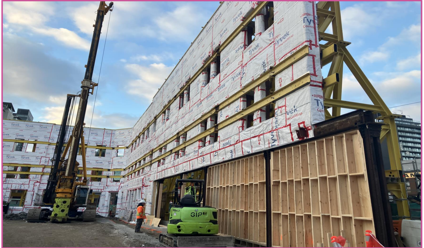
Interior view of works in progress at the North site
