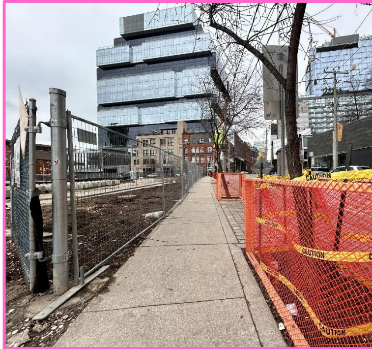
Temporary fencing before noise barriers installation
