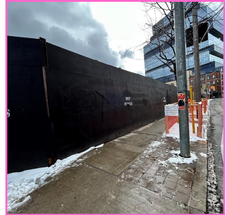
Original hoarding removed
