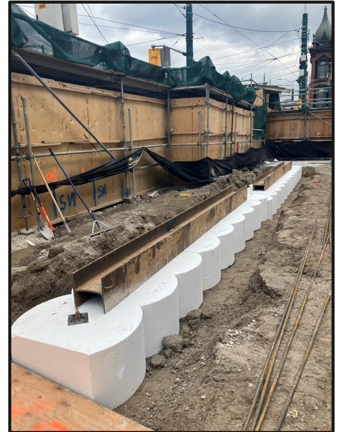
Example of the tops of secant piles
