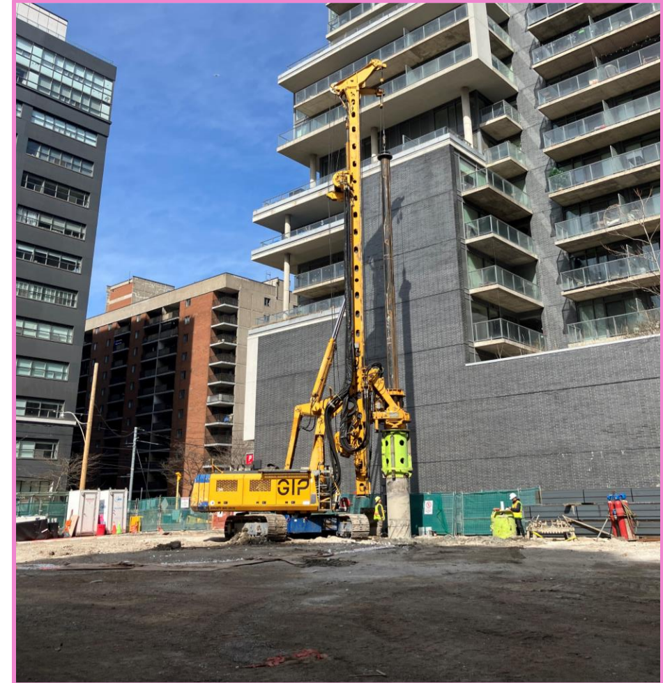
Pile drilling machine at King-Bathurst.
