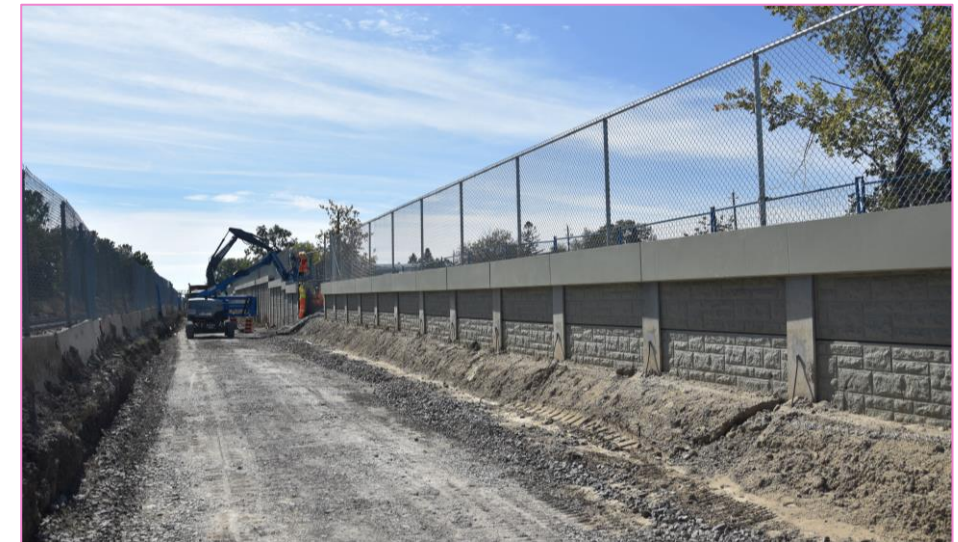
Example of a retaining wall being constructed adjacent to future rails.
