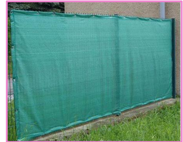
Dust net on temporary fencing.
