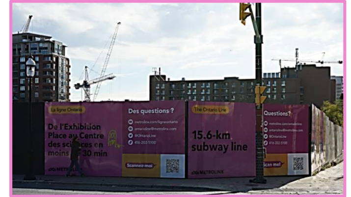
Metrolinx branded hoarding to keep sites clean.
