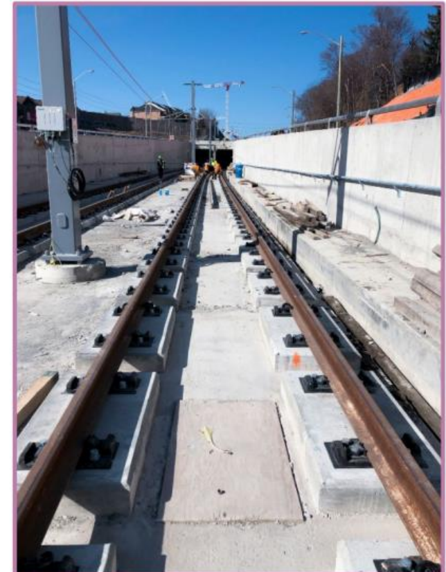
Example of a transit portal
