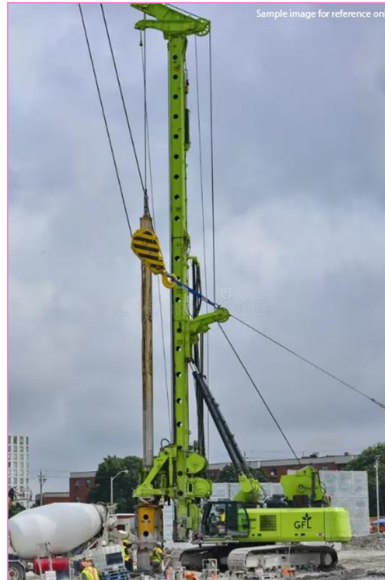
Piling drill rig
