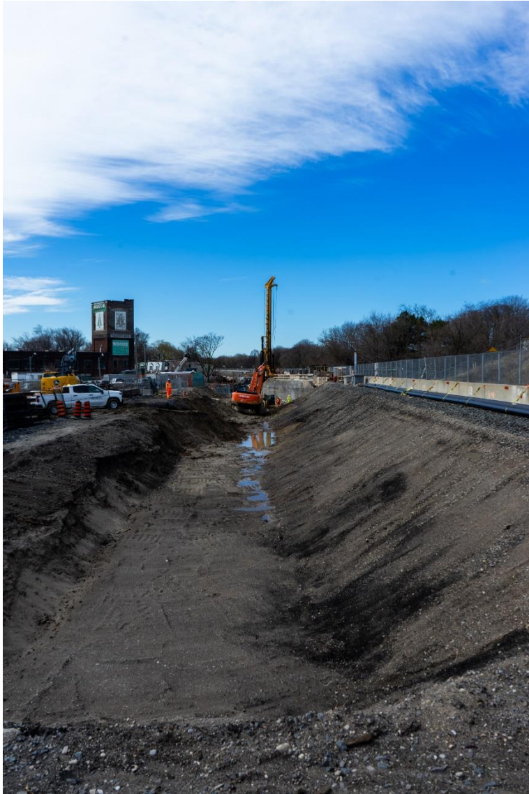
Excavation at Thackeray St looking towards Logan Ave
