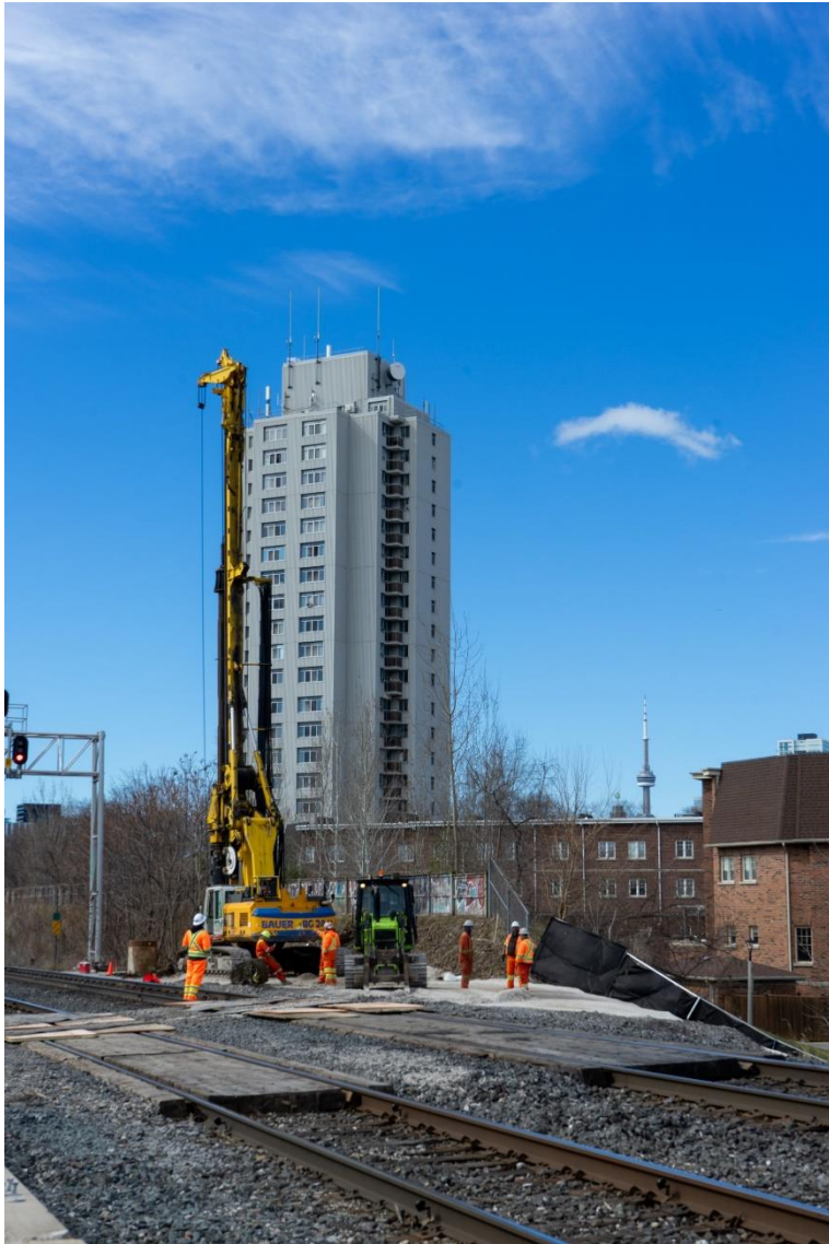
Foundation of new signal bridge being prepared
