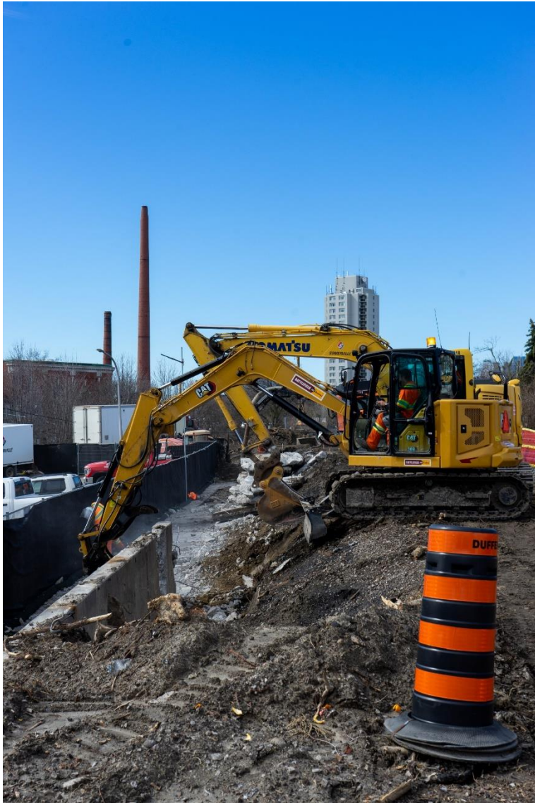
Old concrete retaining wall being demolished
