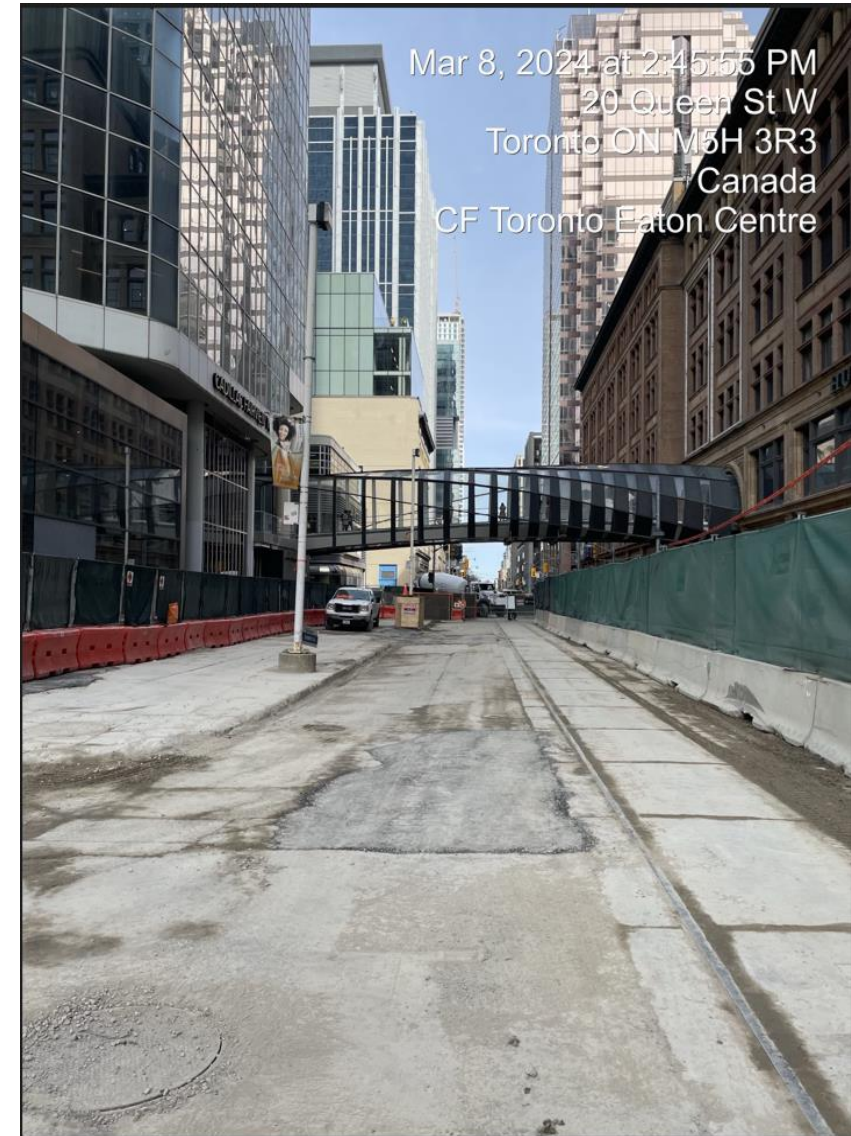
Pedestrian bridge at the CF Toronto Eaton Centre
