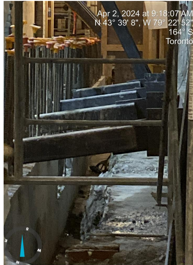
Bracing to support existing basement wall during construction
