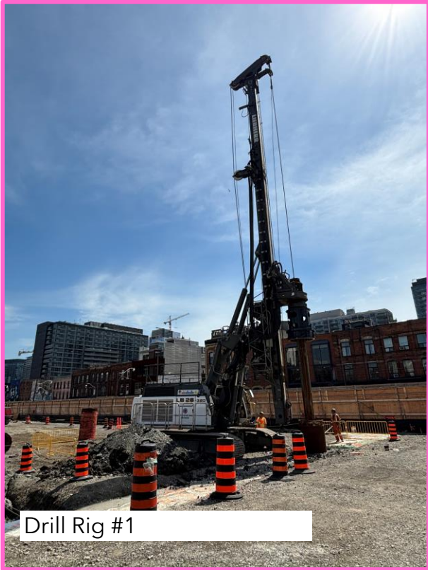
Installing Casing
