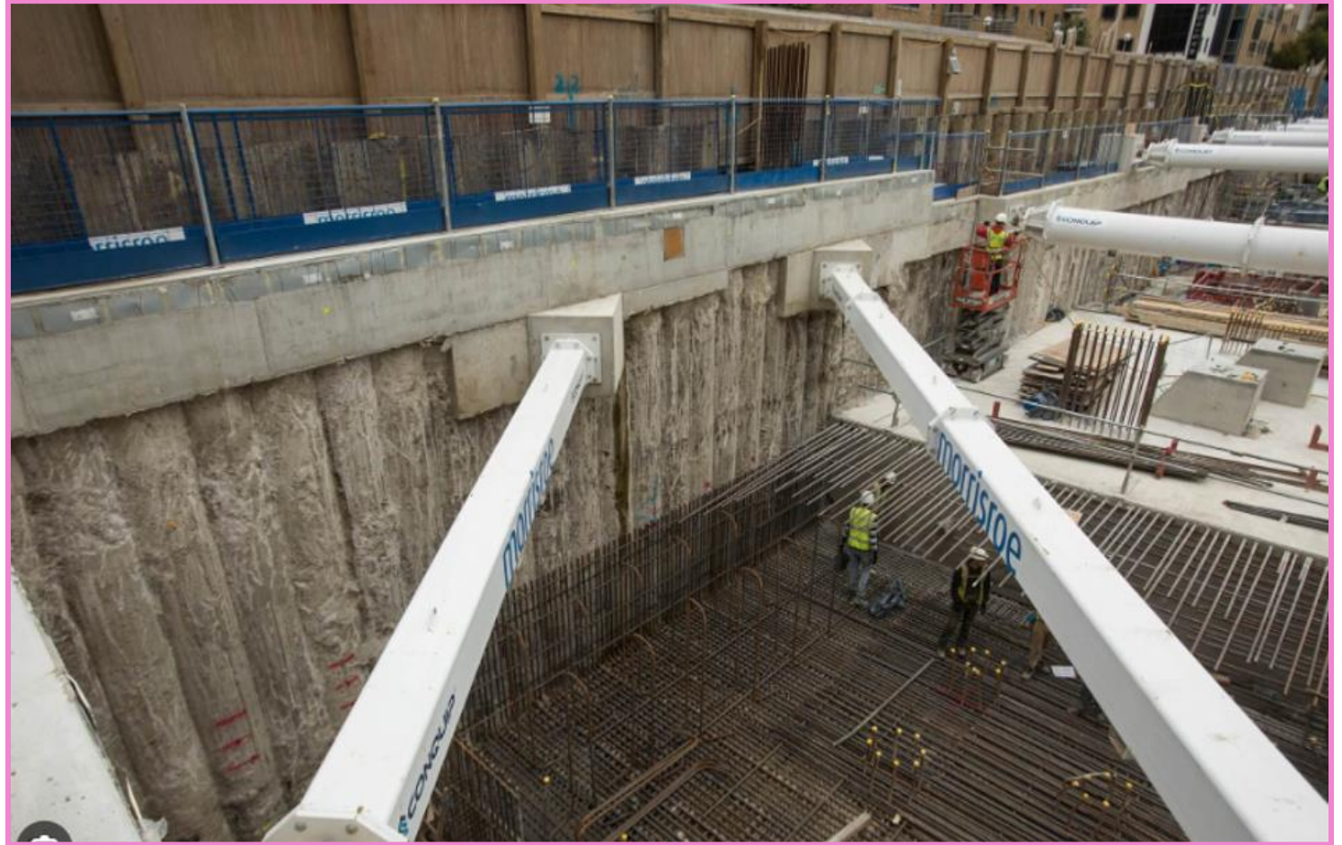
Example of secant pile wall
