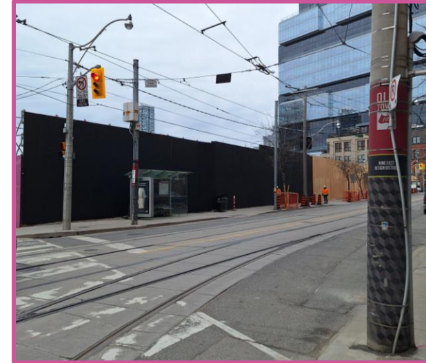
Example of 5m high hoarding / noise wall
