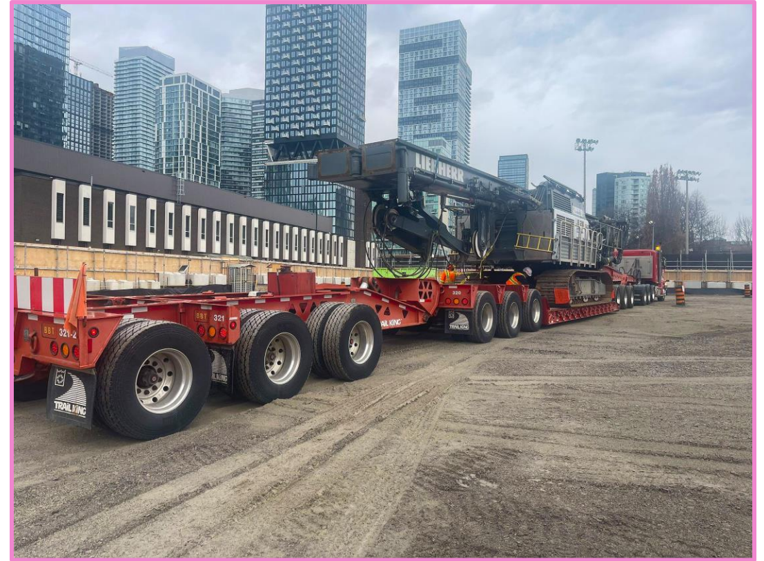
Example of a drill rig delivery
