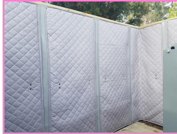
Sound dampening blankets placed on the inside of site hoarding.
