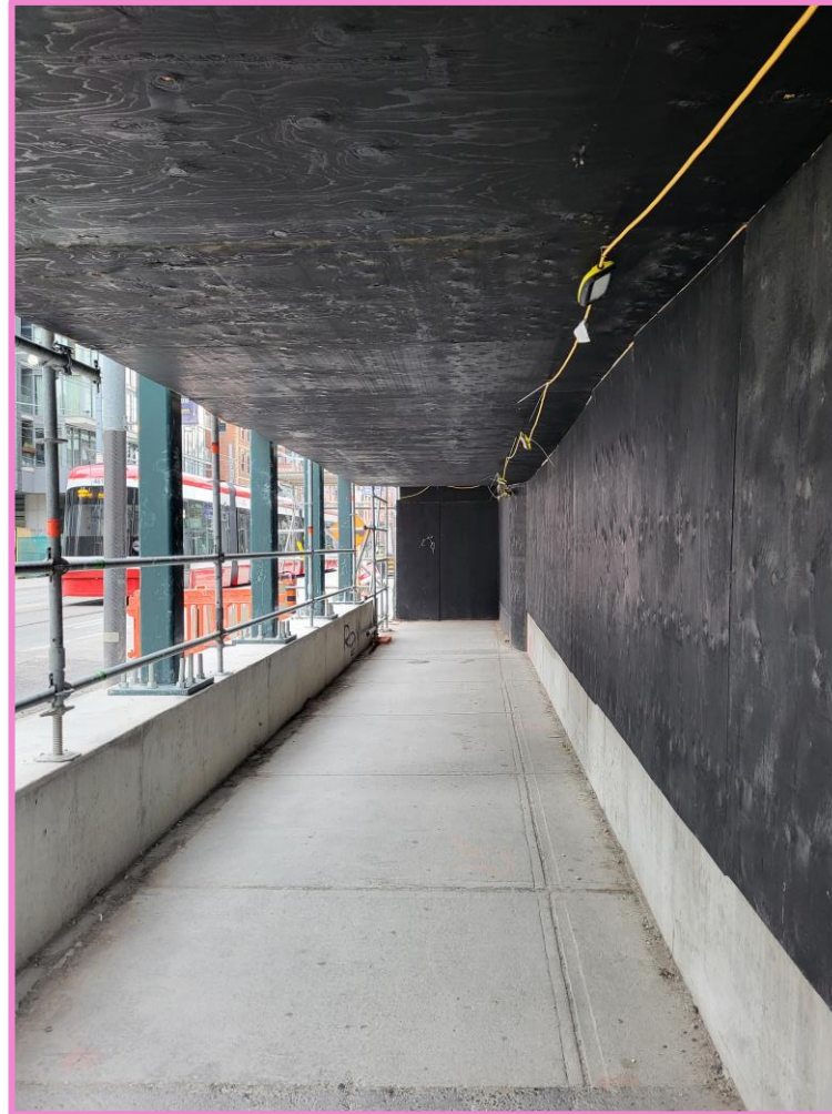
Installation of long-term hoarding on the south site, and fast fence on the north site.
