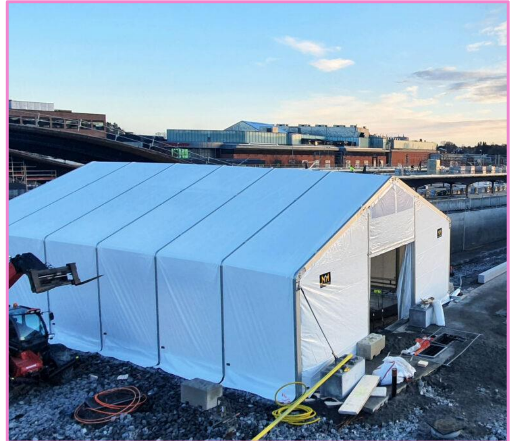
Example of an acoustic shelter tent, to protect from noise, dust and weather during excavation.
