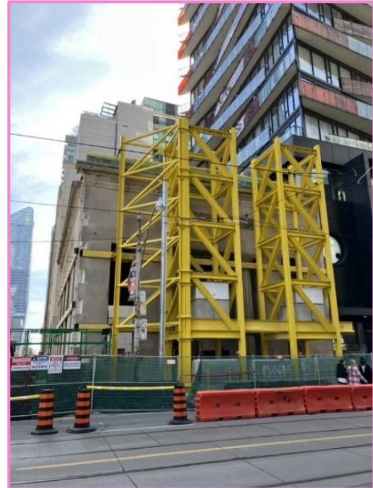
Façade retention work at the south station
