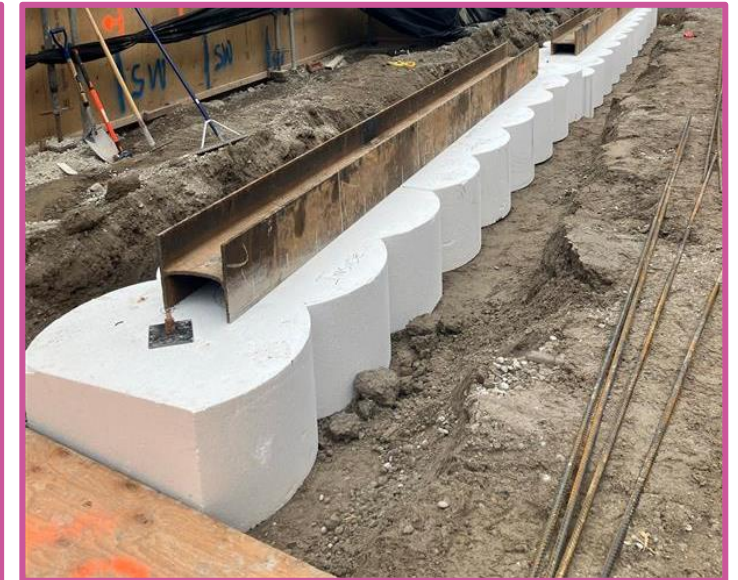
Typical example of guide wall installation to properly align the secant piles for installation.
