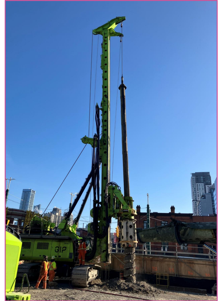
Drilling machine used in pile construction
