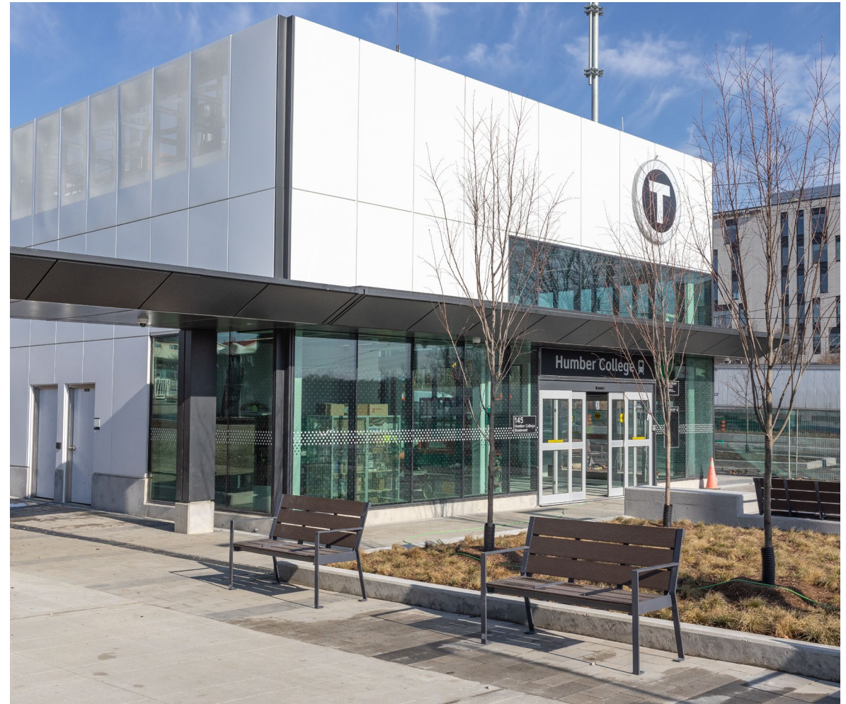
Photo: Humber College station, South building external view. 2023.11.30
