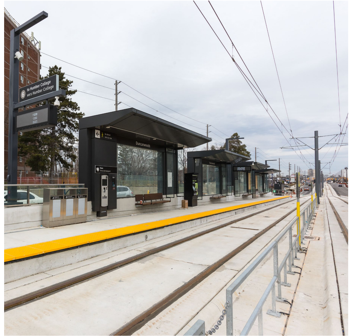
Photo: Duncanwoods stop westbound platform, northeast view. 2024.03.28
