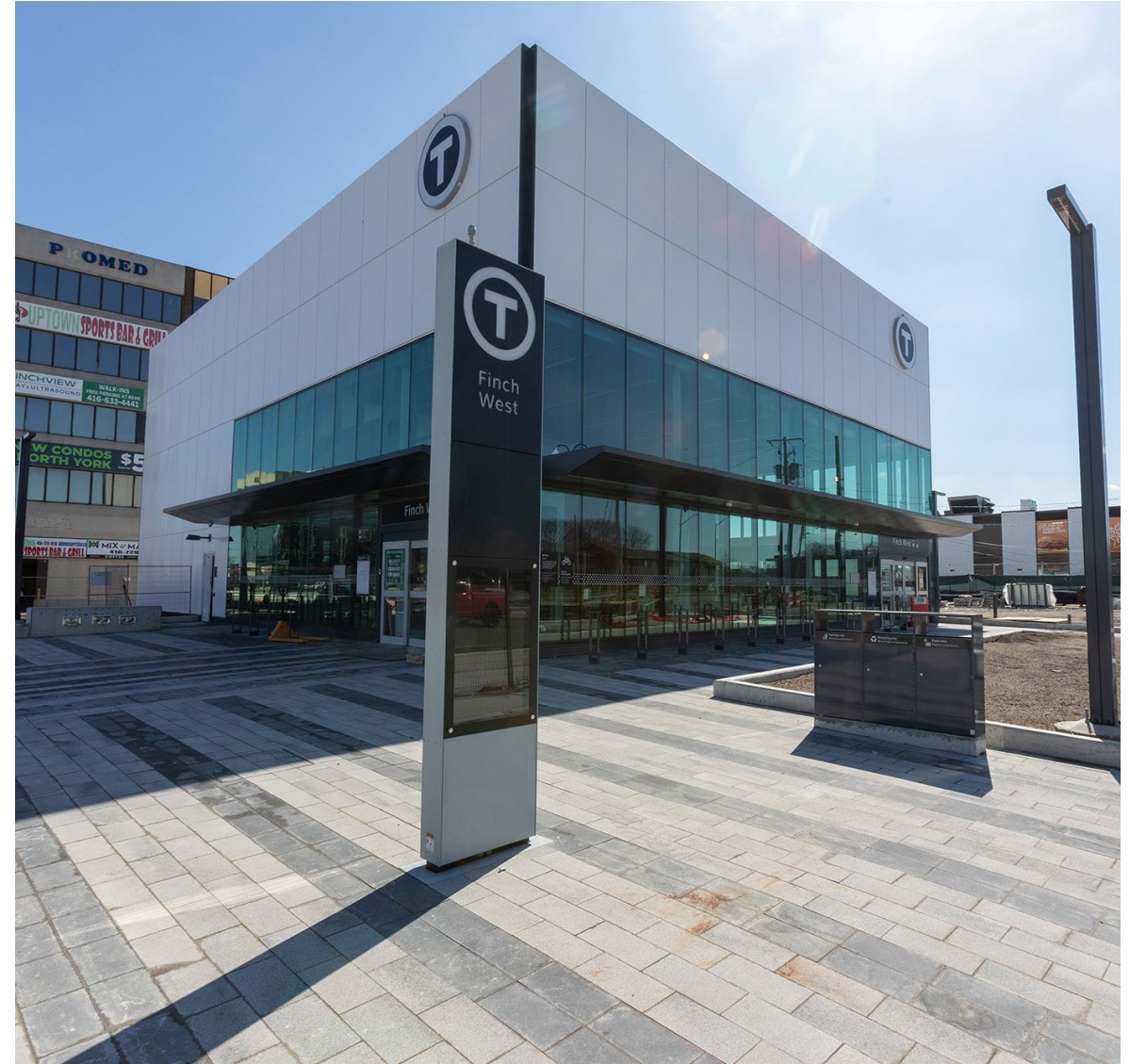
Photo: Finch West station southeast view. 2024.03.28
