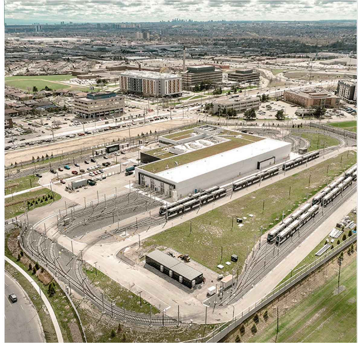
Photo: Maintenance and Storage Facility northeast aerial view. 2024.03.24
