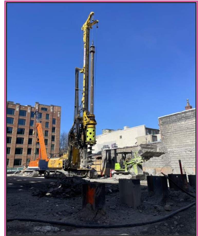
View of piling drill
