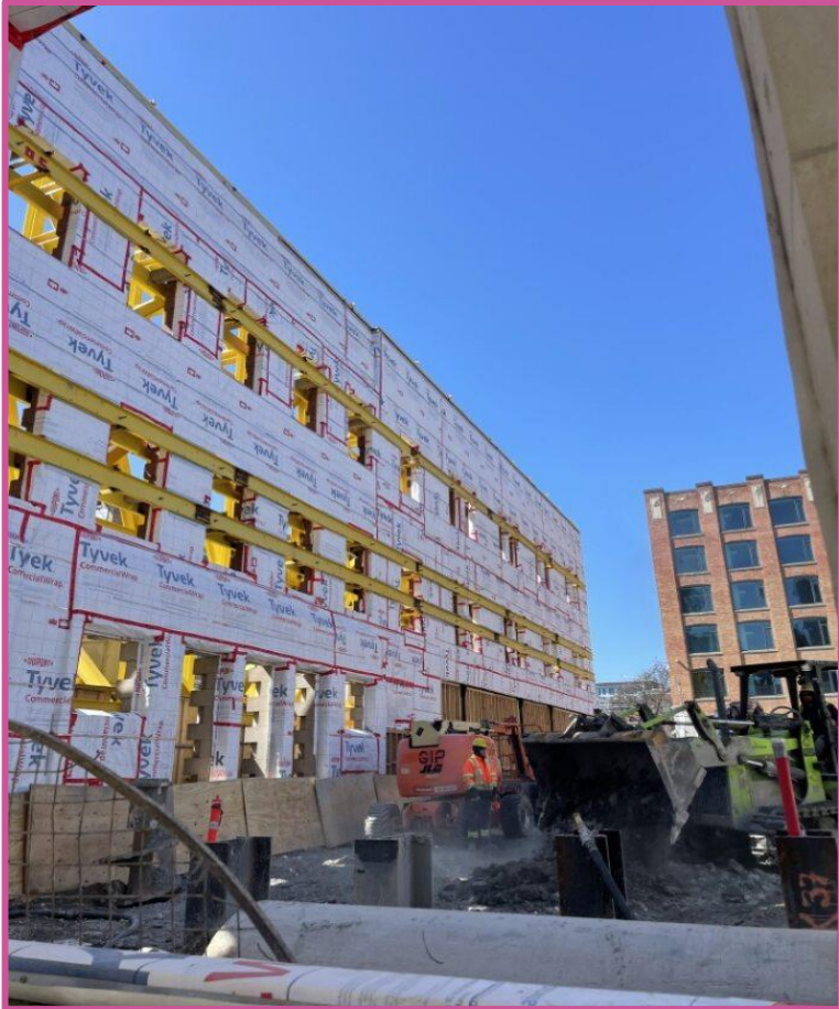
Interior site view of retention towers
