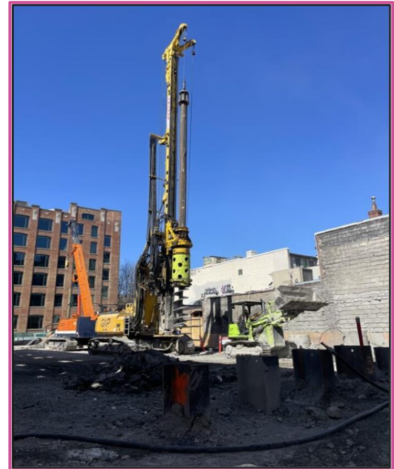
View of piling drill
