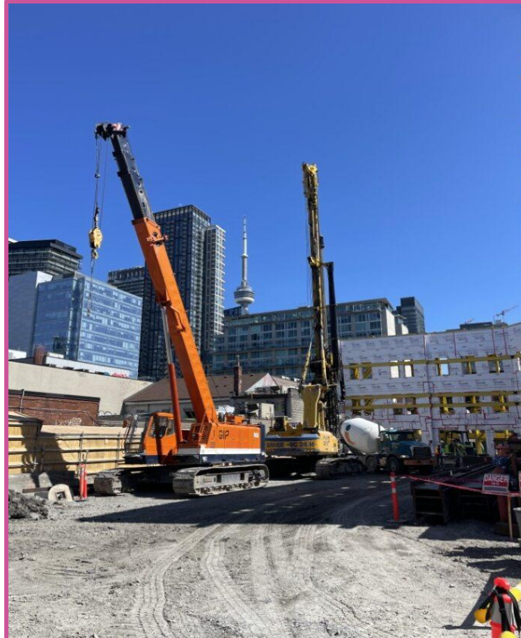
View of crane onsite, used to support pile drilling
