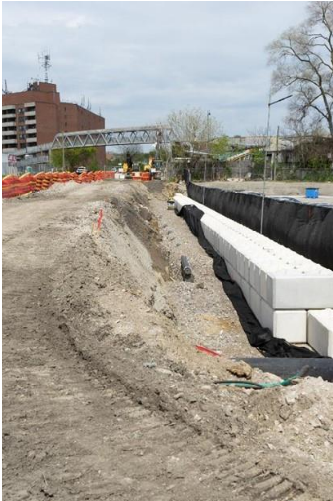
Pre-cast concrete blocks being installed by the LCBO.
