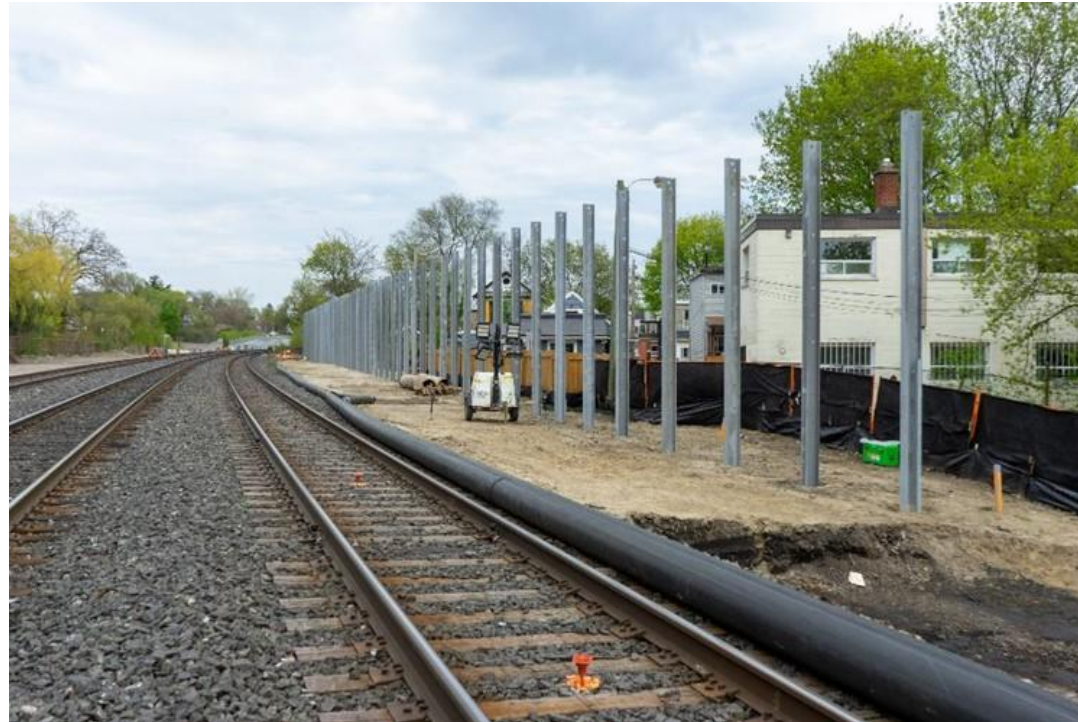
Steel piles installed by Galt Ave. These will support noise barriers.
