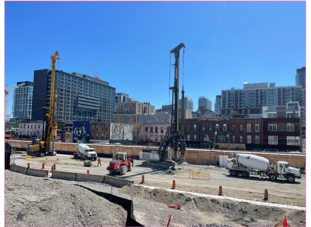
View of piling work zone
