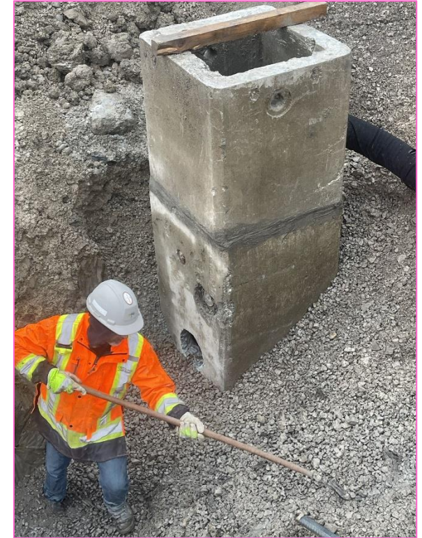
Backfilling drainage structures
