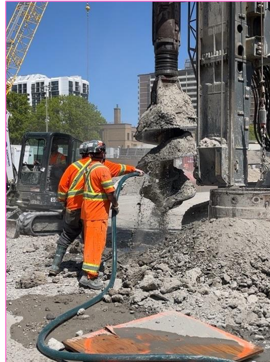
Water sprayed on dry spoils to reduce dust
