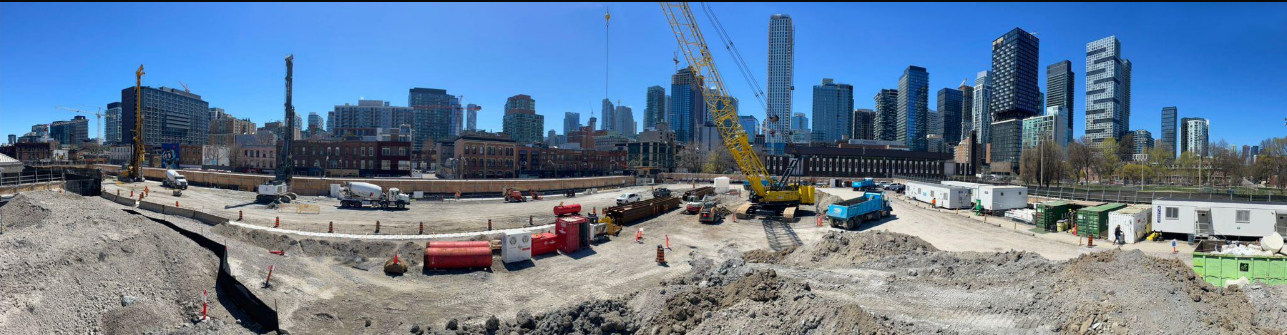
Panoramic view of the piling work zone looking south
