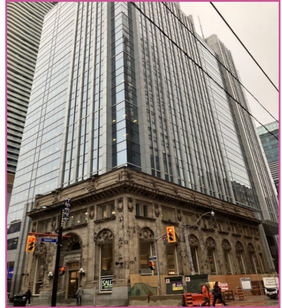
2 Queen Street East building as of April 11, 2024
