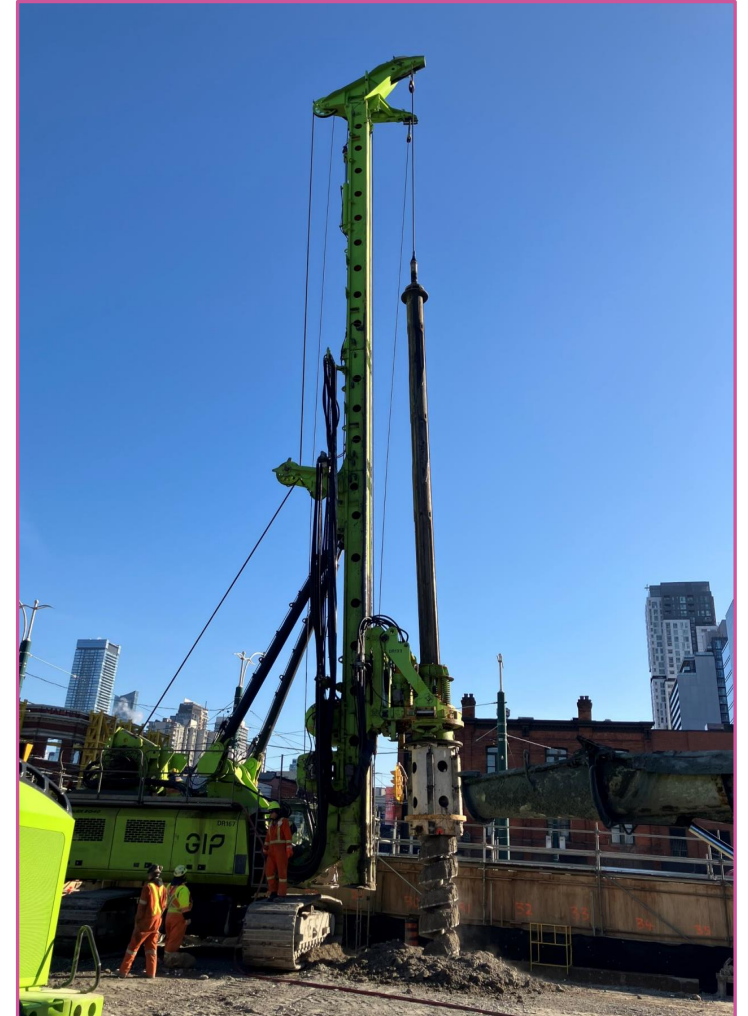
Drilling machine used in pile construction
