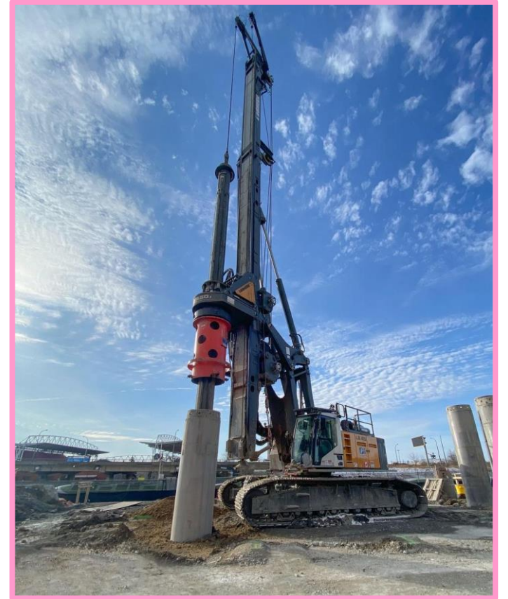
Piling machine from another Ontario Line project
