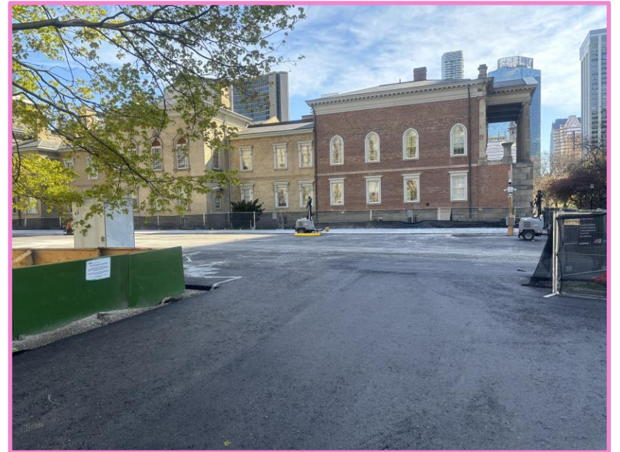
Laydown area with asphalt paving at the North site.
