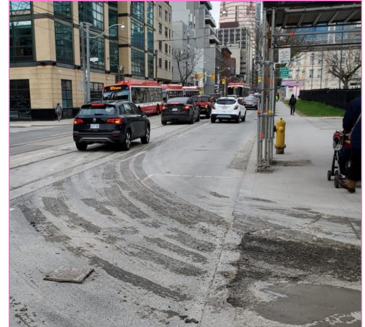
Dirt and mud tracked out from the construction vehicles
