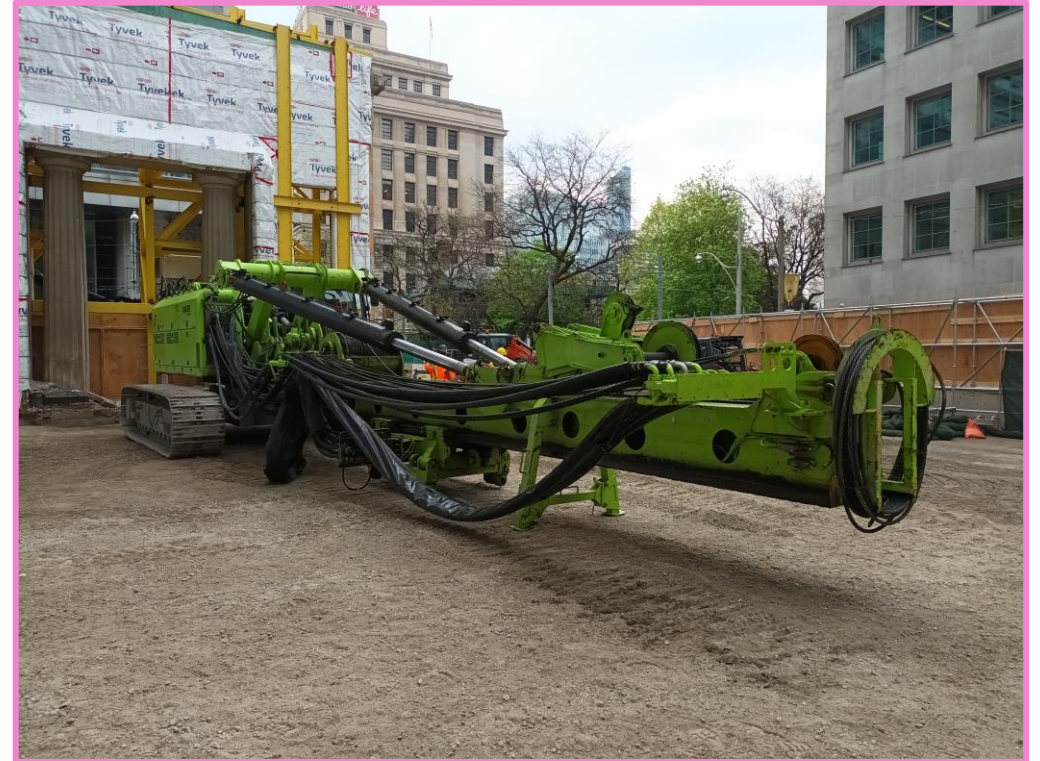
Image of pile drill rig at the South site.
