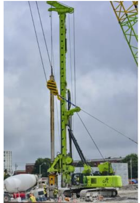
Pile drilling rig shown above
