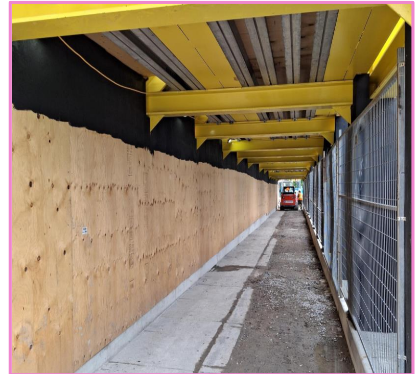
View of the overhead protection at the future North station site as of May 28, 2024
