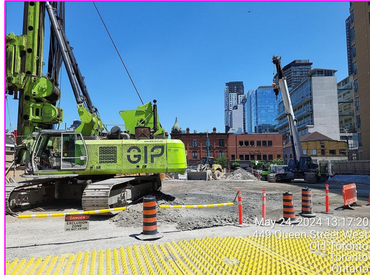
View of the future South Station entrance as of May 24, 2024.
